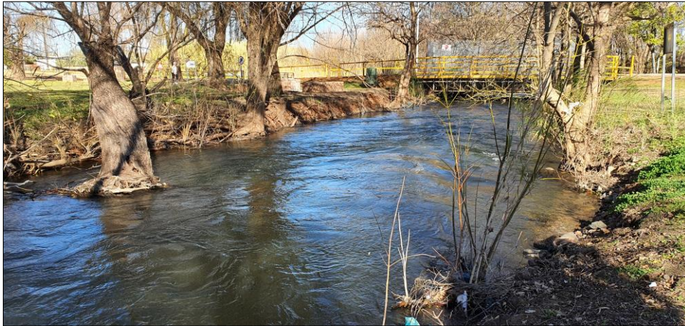
Figure 9: General view of survey footprint (Mooi River with unstable bridge)
