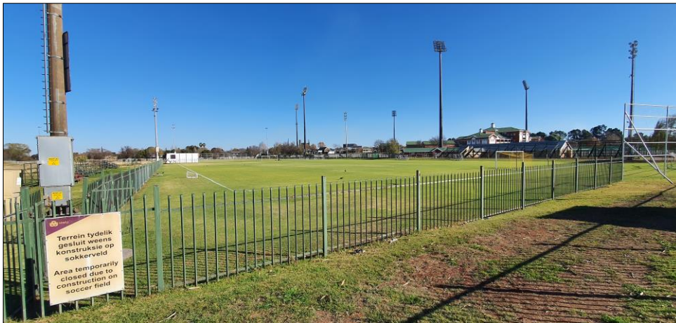
Figure 17: General view of the existing infrastructure in the area
