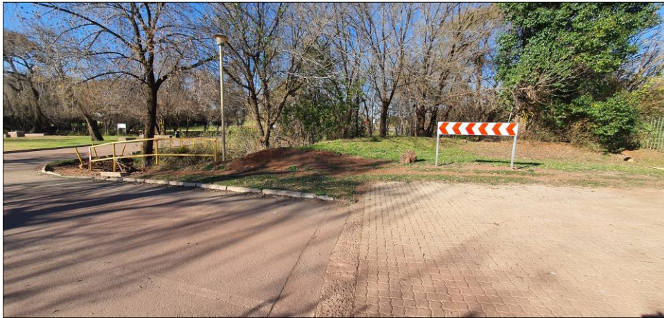
Figure 16: General view of the location of the new road and bridge
