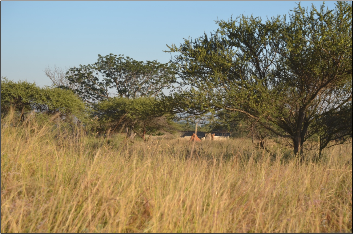
Figure 11. Old concrete dam on site
