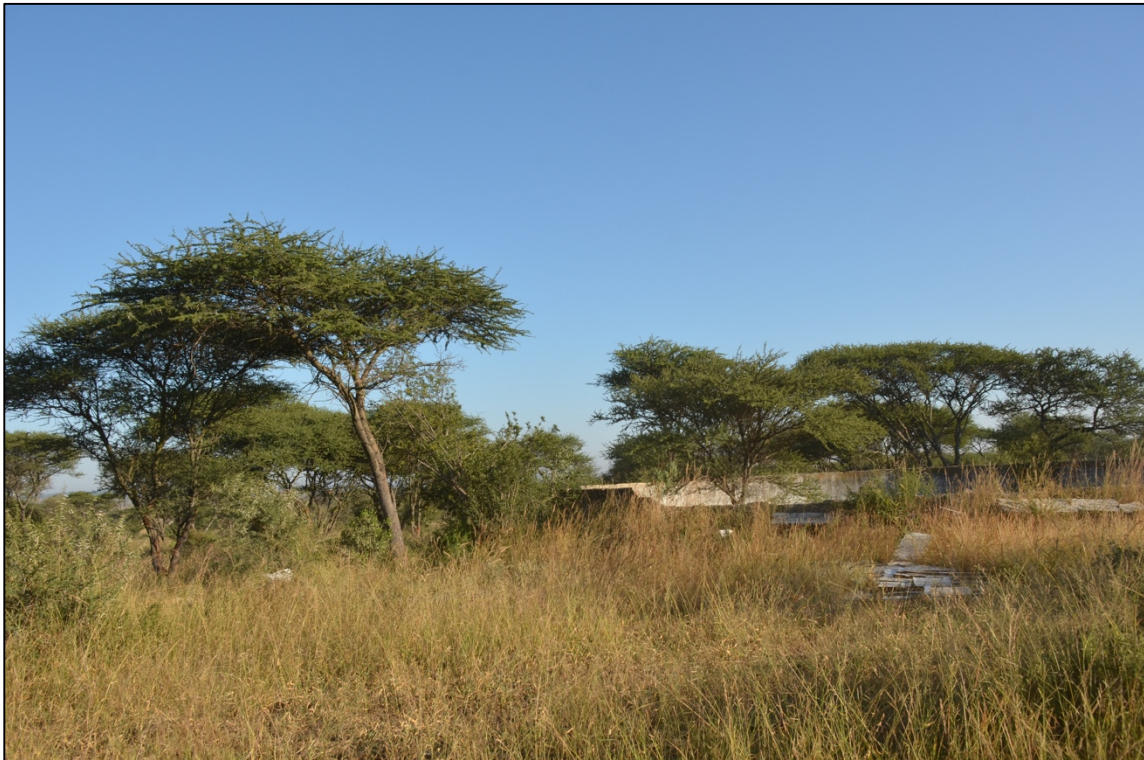
Figure 18. Dilapidated cement dam on site
