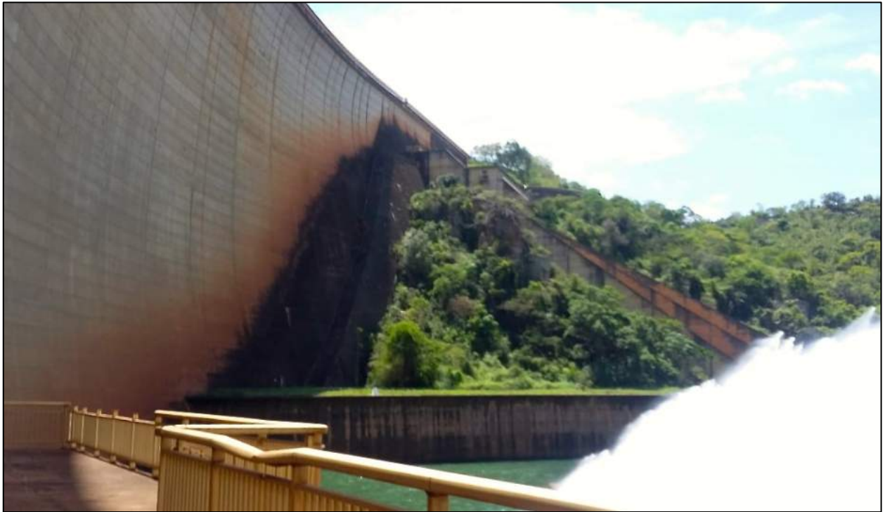
Figure 13. Pongola Dam Wall
