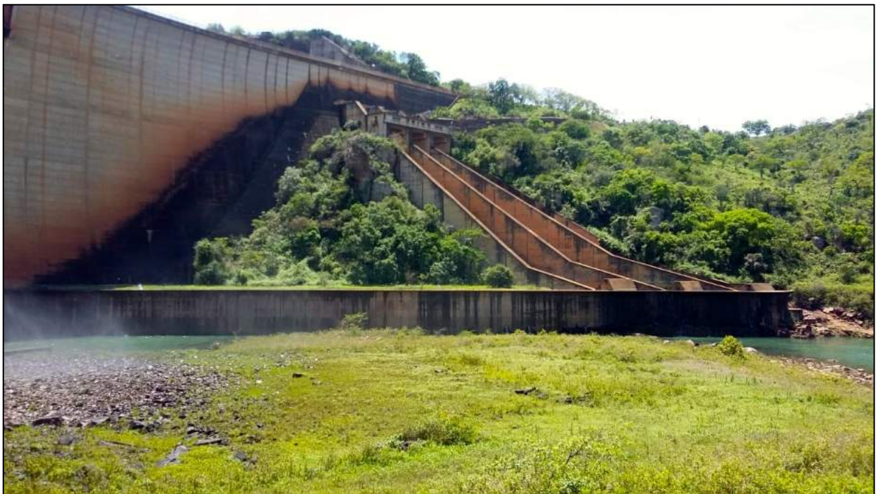
Figure 12. Pongola Dam Wall
