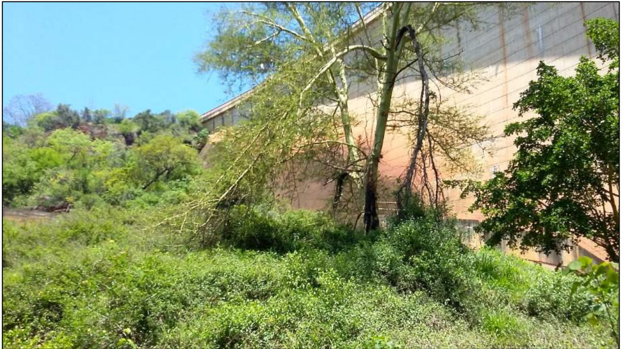
Figure 8. Pongola Dam Wall
