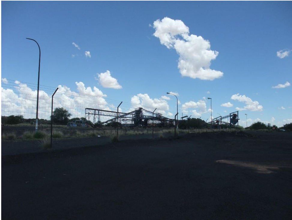
FIGURE 11: OLD INFRASTRUCTURE IN THE SURVEYED AREA.
