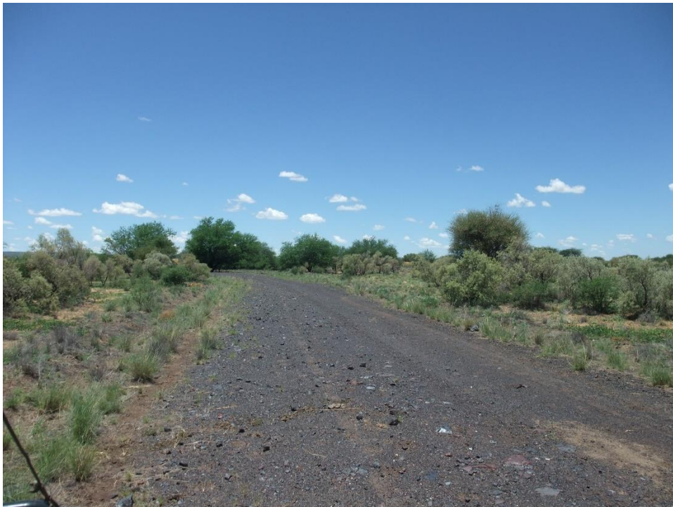
FIGURE 12: GENERAL VIEW OF THE SURVEYED AREA SHOWING A GRAVEL ROAD.
