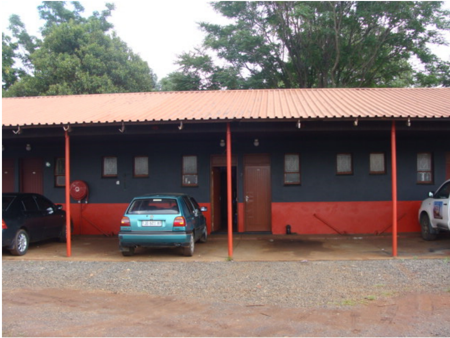
Figure 14 Some of the rooms of the hotel, dating to the 1960's/ 70's.
