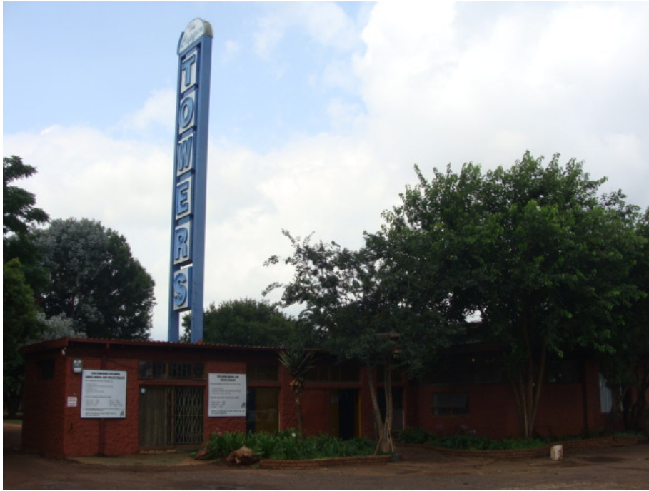
Figure 12 Main building of the Towers Hotel. Note changed made recently to the structure.
