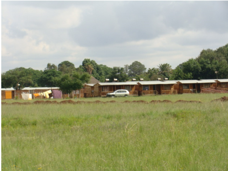
Figure 16 Recently added rooms to the hotel, some being non-permanent structures.
