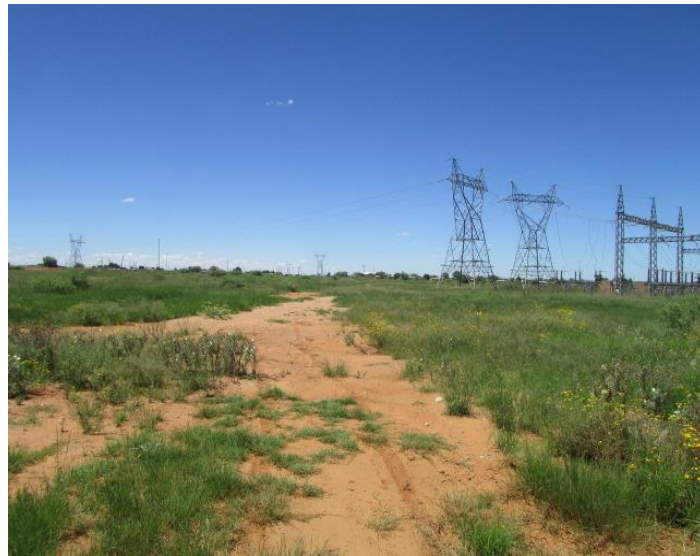
Fig.9: ESKOM powerlines traverse sections of the area.
