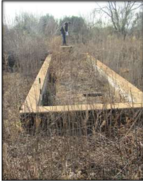
Fig.21: Another water trough at Site 2.
