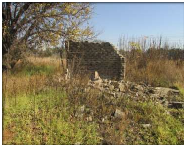
Fig.14: A view of the Site 1 structural remains.
