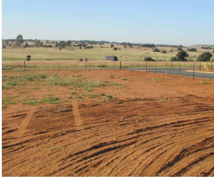
Fig.5: Parts of the area has been scraped and leveled & the whole study area has been fenced-in.
