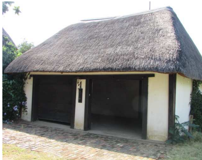
Fig.12: The garages of the above homestead.
