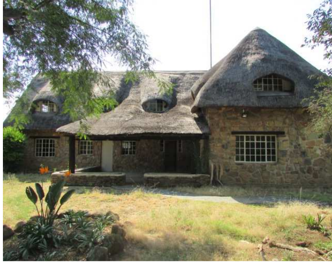
Fig.13: The front view of the homestead.
