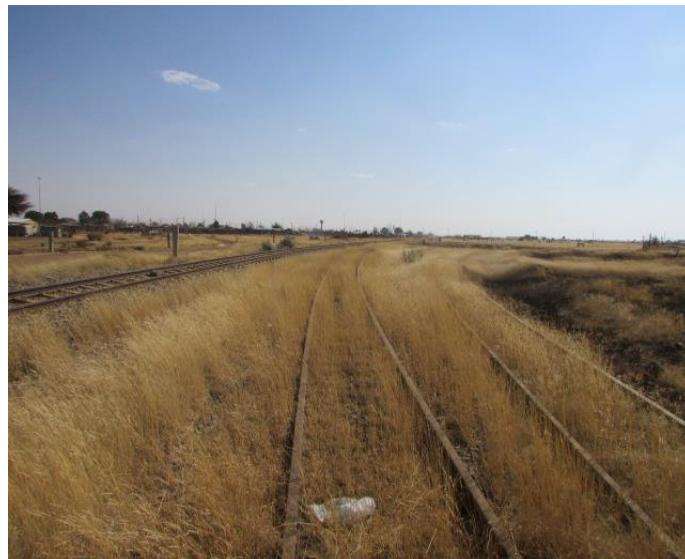
Fig.7: Another section of the railway line.
