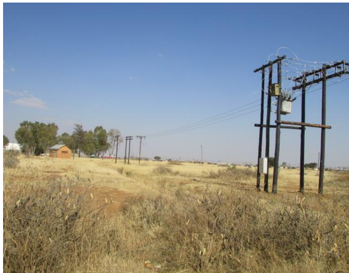
Fig.10: Some telephone/powerlines traversing the area.
