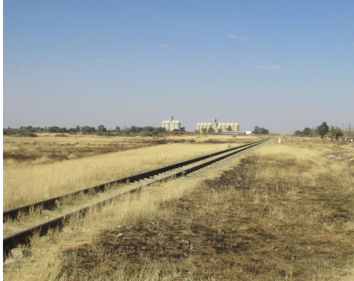
Fig.6: A view of a section of the railway line towards the silos.
