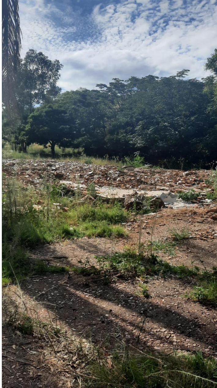
Figure 14: All the recent structures identified have been reduced to foundations and rubble.
