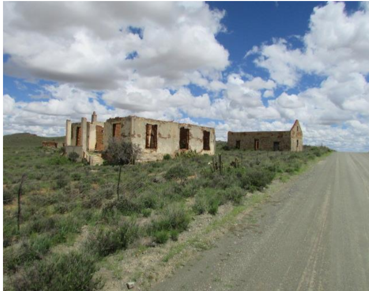
Fig.37: Ruins of old farmstead near Burgerville Site 35.
