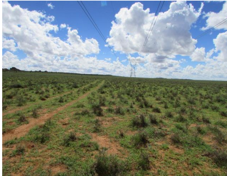
Fig.11: View of one of the ESKOM powerline corridors close to the Area 1 proposed substation.
