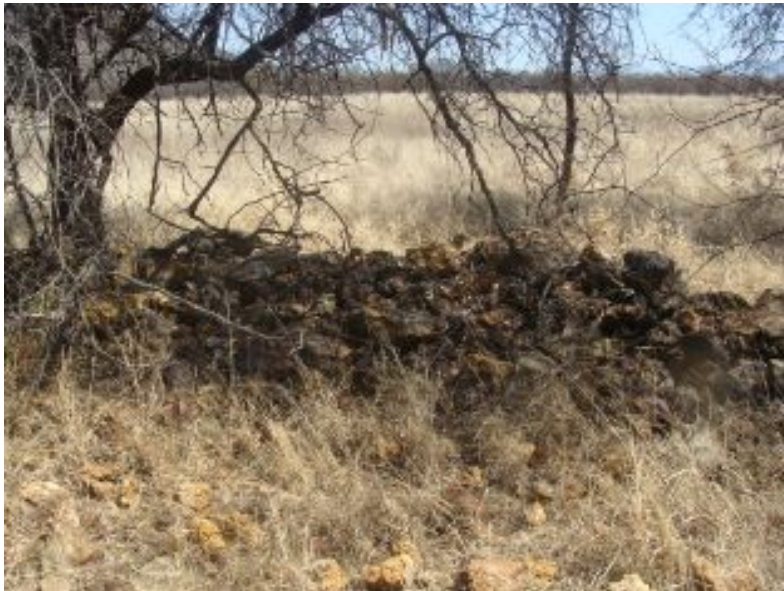
Figure 16: Foundations of stone and cement structure.
