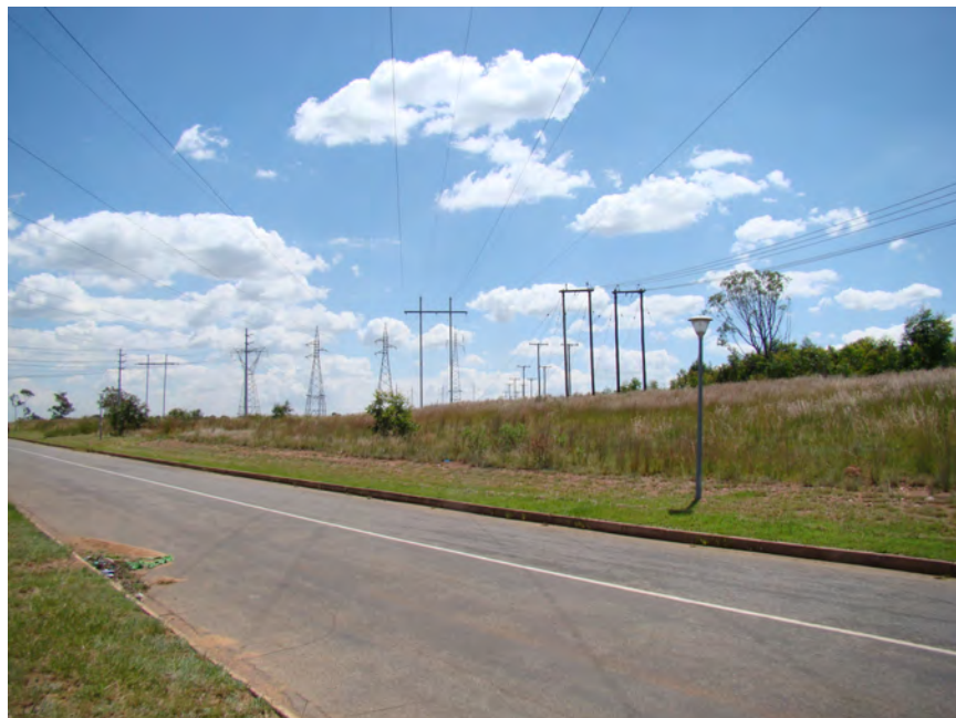
Fig. 28: The existing lines from the Middelburg substation, facing west.
