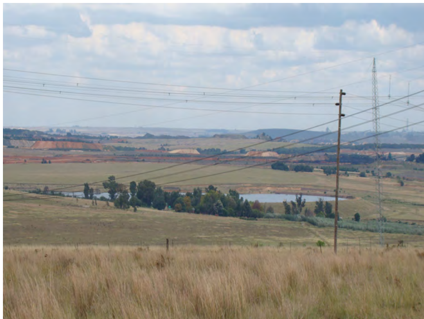
Fig. 20: View from the north towards the proposed B MTS substation in the south. The view of this area from a distance, show the highly disturbed section with cultivated land as well as coal mining activity.
