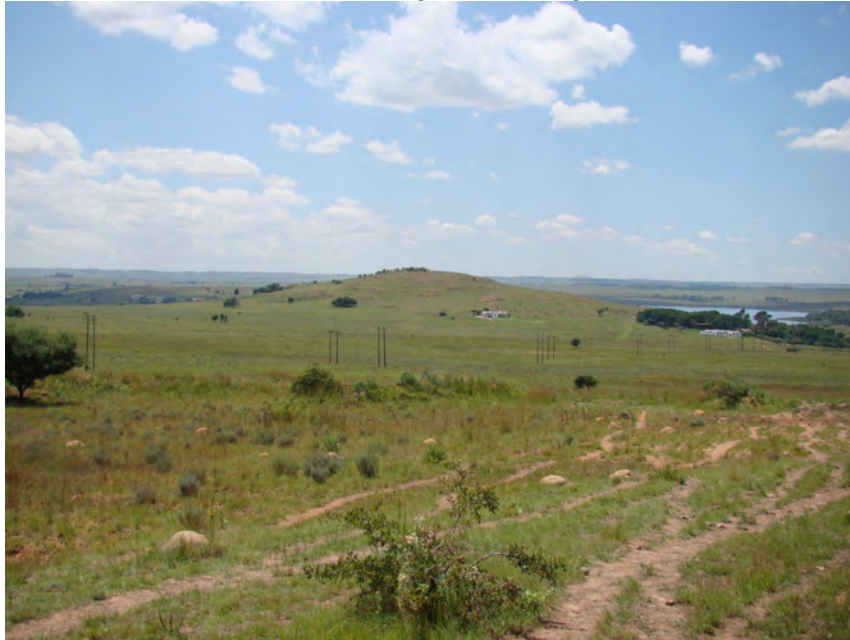
Fig. 1: Route Option 1 & 2: A – D: View from Doornpoort substation (A) towards hill (D). The existing power lines are visible and the proposed line will run along these lines. It is recommended that these lines be upgraded. The smallholdings are utilized for small scale farming and cattle grazing.
