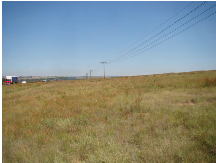
Fig.6: D - E: The existing lines run parallel with the N4. It is recommended that the lines be upgraded from D until passes the Heritage 1 features in order to avoid impact on this feature. The lines are approximately 40m from the feature towards the north. Game farming is one of the activities in this section.
