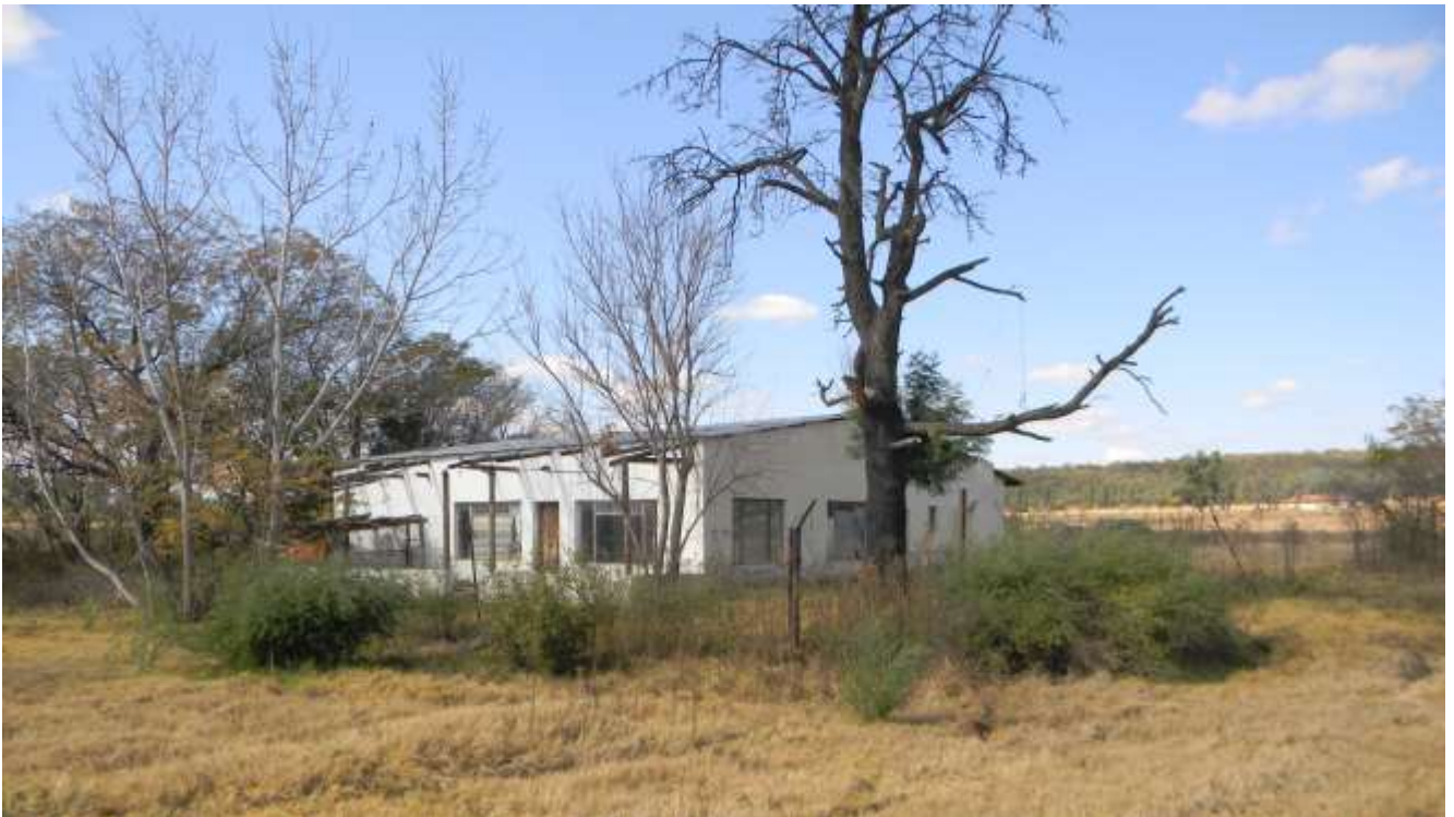
Plate 37: Photo 37: Showing a historical farm building (Photograph © by Author 2021).
