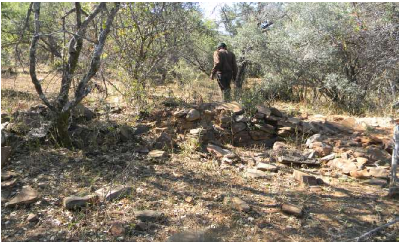
Plate 33: Photo 33: View of a farm owner showing the collapsing structures (Photograph © by Author 2021).
