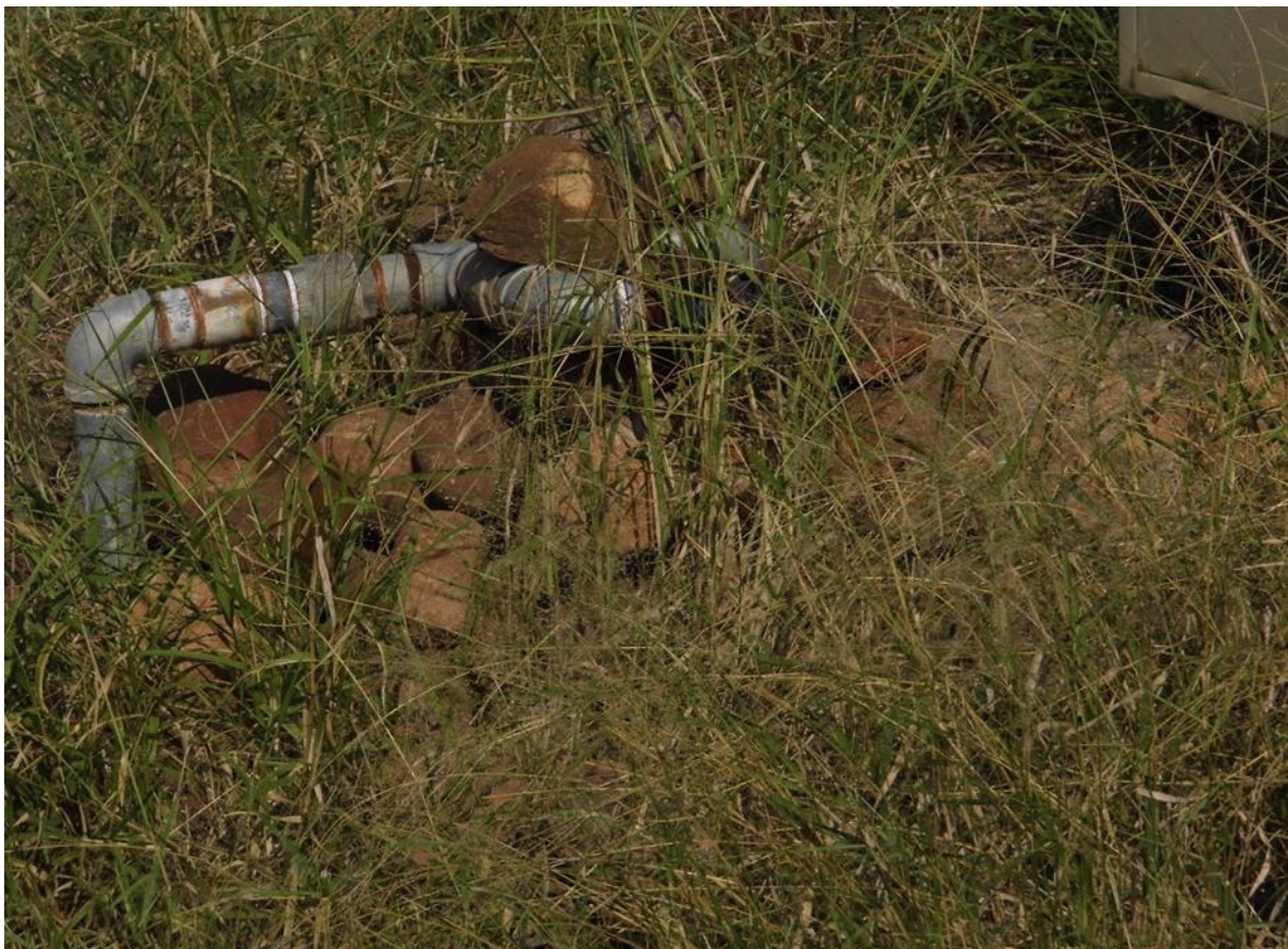
FIGURE 11 THE EXISTING BOREHOLE
