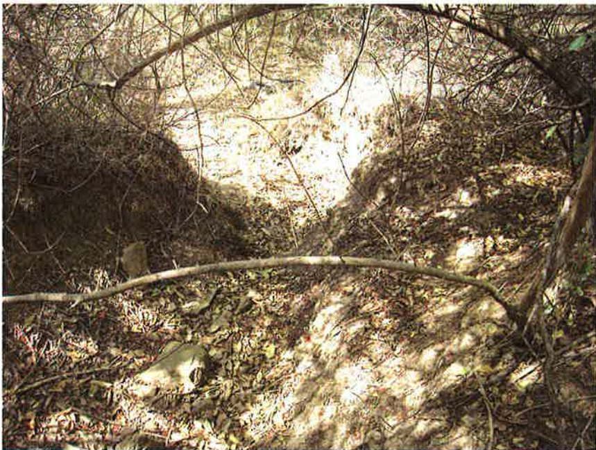
Erosion - waterway. S 29° 50' 12,0" and E 30° 57' 25,6".
