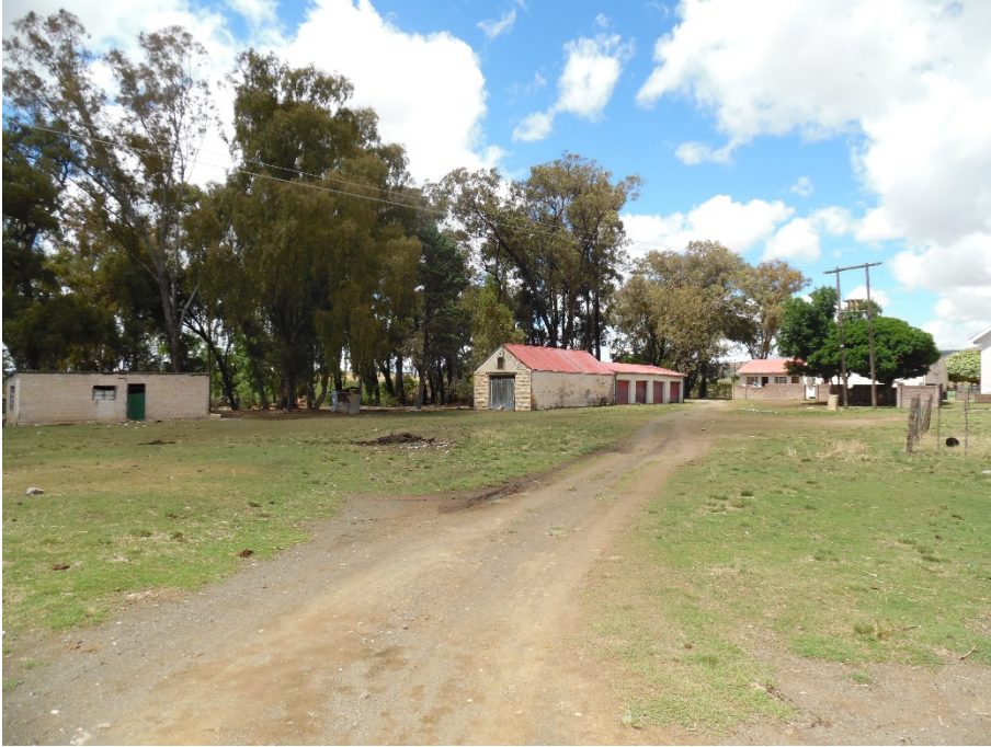
Photograph 9: Structures situated to the north of main residence
