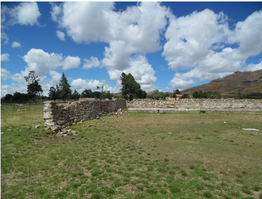
Photograph 8: Animal enclosure structure
