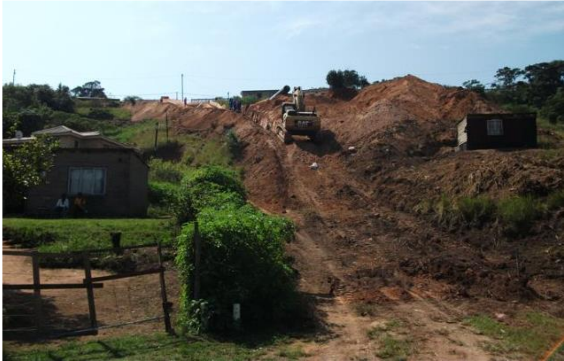
Figure 7: Excavations for water pipeline
