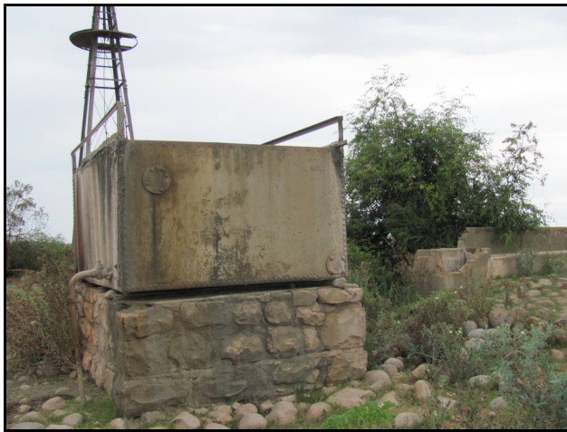
Plate 11: Dressed stone base with cast iron water reservoir.
