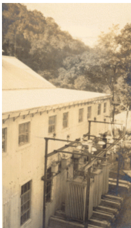
Transformers at the Sabie Gorge Power Station
