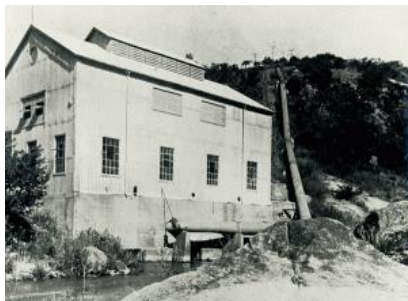
The Sabie River Gorge Power Station
