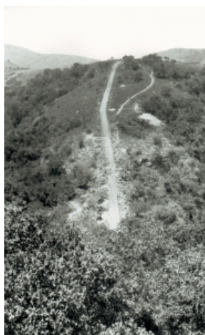
Pipeline at the Sabie Gorge Power Station
