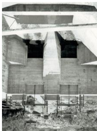
Setting basin at intake Works
