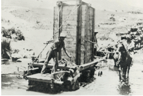
Transport of a Siemens transformer.
