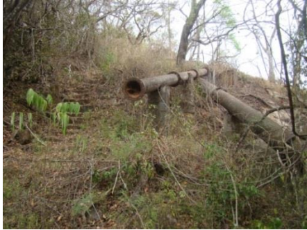
Fig. 5: The staircase and pipeline which channeled water to the Hydro.
