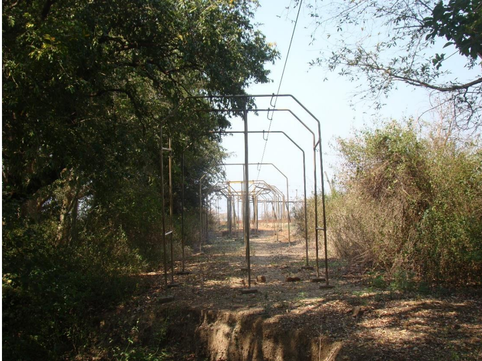
Fig. 14: Farm infrastructure is visible in some sections.
