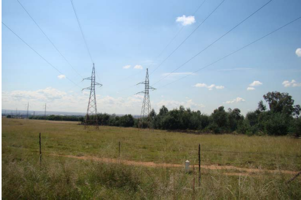
Fig. 11: Point G on the ESKOM map: This is where the proposed line will link up with the existing Athlone line.
