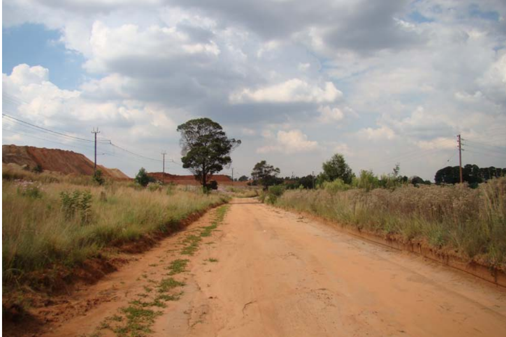
Fig. 3: Point E. The current coal mine is visible to the left as well as the railway line, servitude, SASOL gas line and service road. This is where the proposed line will follow an easterly direction, along the railway line to point F. Existing power lines are visible to the right.
