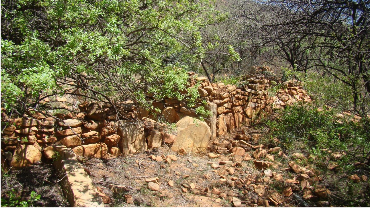
Fig. 13: The foundations of the historic farmhouse.
