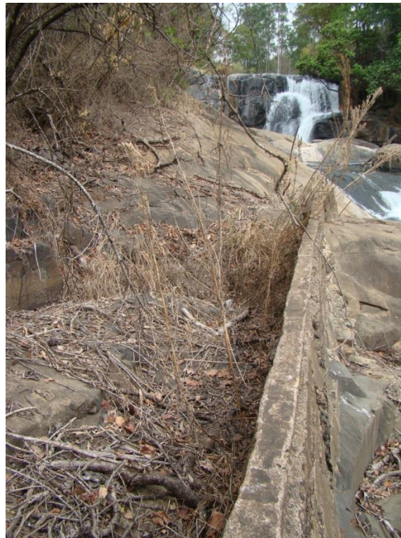
Fig. 13: The concrete wall of the holding pond is still visible.
