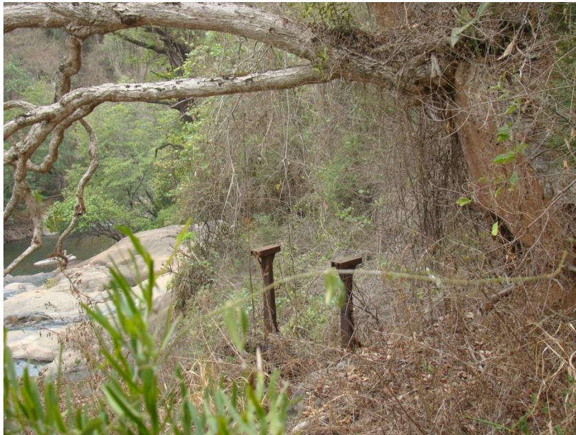
Fig. 15: Metal supports which were used for the original Hydro Power station are still visible.
