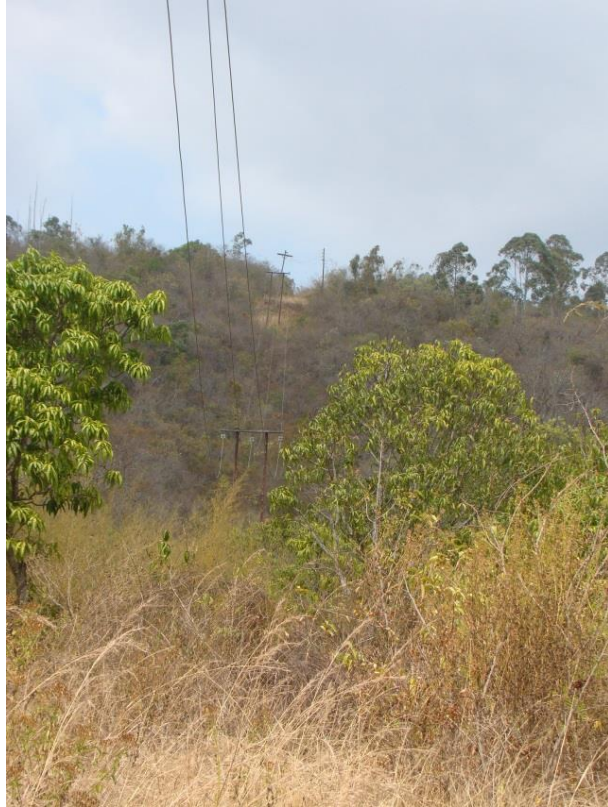
Fig. 18: Power will connect up to the existing powerlines approximately 1km from the hydro building. Sections of the 11Kv powerline will be below ground and other sections above ground.
