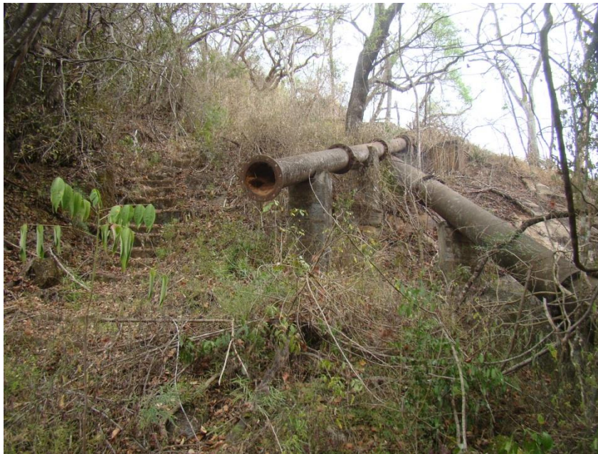
Fig. 11: The staircase up to the holding dam is visible on the left, with the pipeline which supplied the water to the power station.
