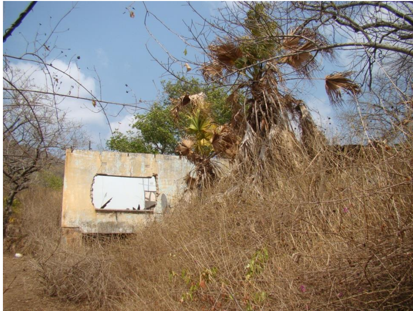
Fig. 20: The ruin of the previous farmhouse.
