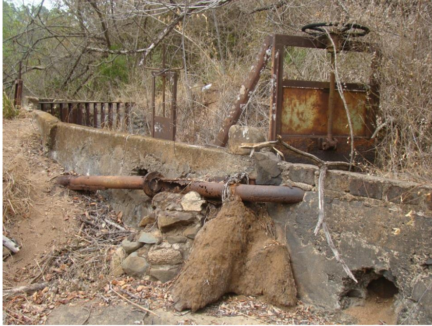
Fig. 12: The holding pond above the power station which supplied the water to the power station.
