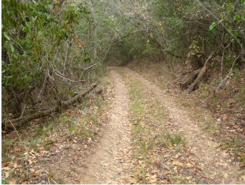
Fig. 8: The existing access road to the hydro building will be stabilized (less that 5m in width).
