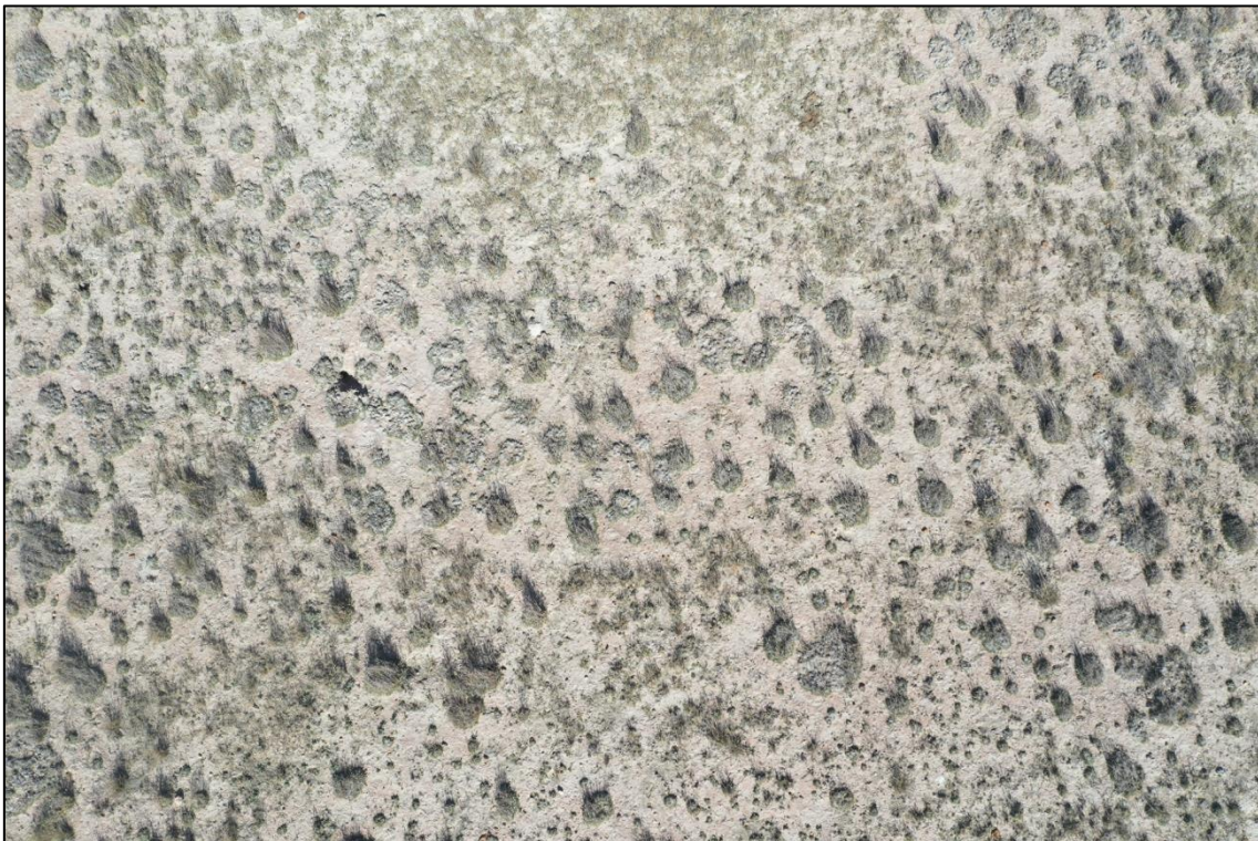
Figure 30. Aerial Survey of the Study Area
