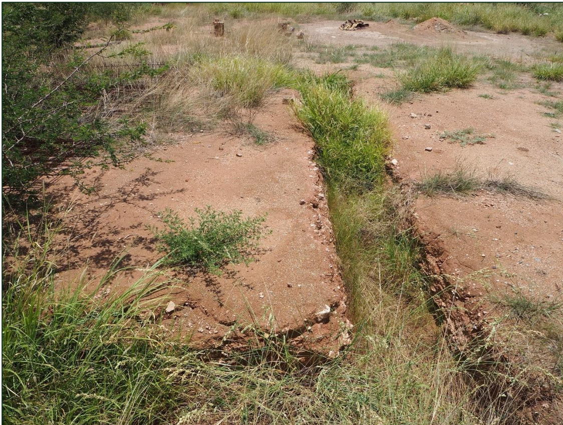
Figure 48. Finished foundation excavations
