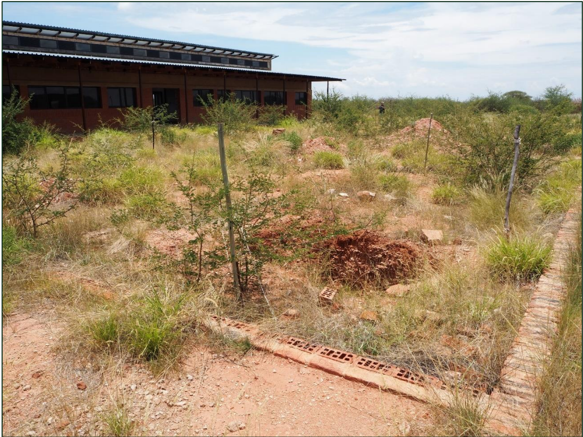
Figure 46. Foundations of structures still to be finished
