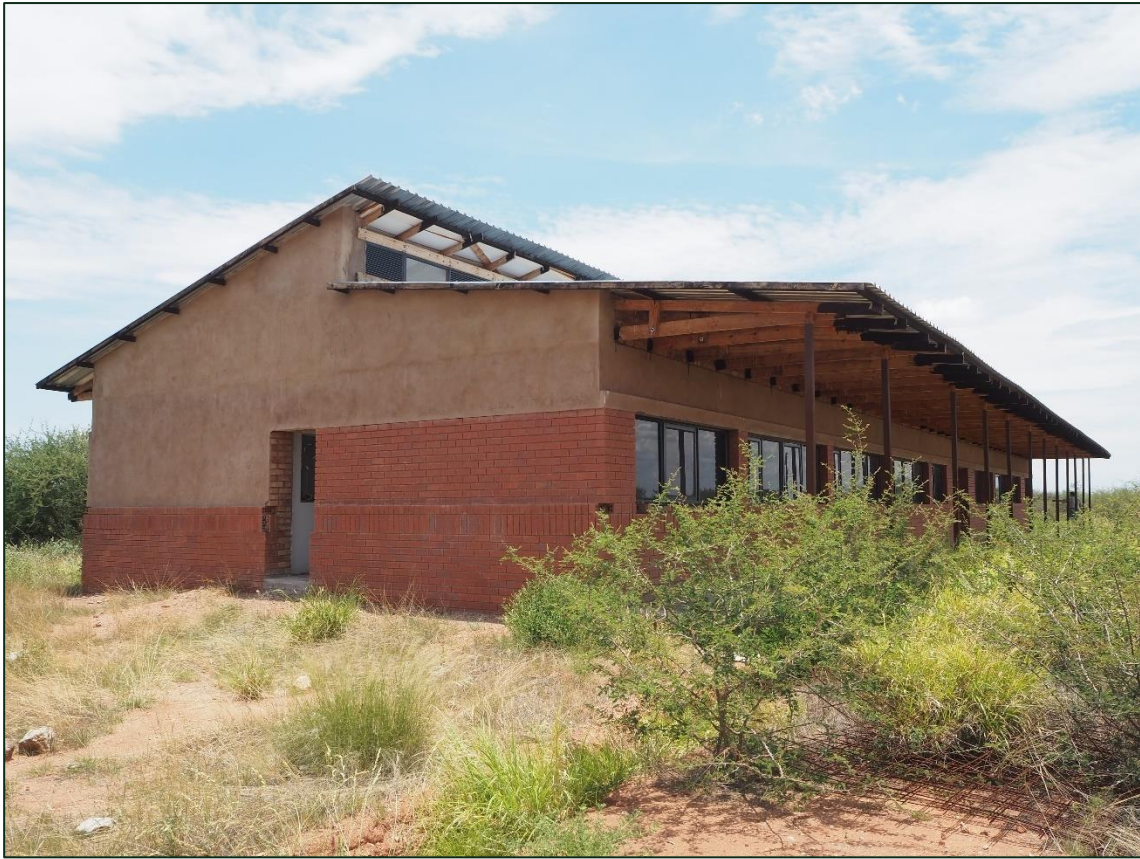
Figure 45. Largely finished Office Complex structures
