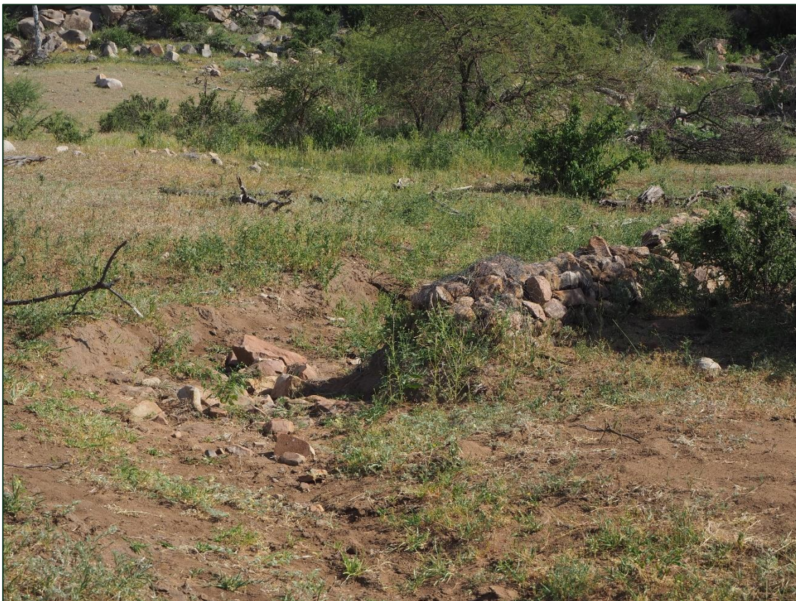
Figure 72. Secondary erosion as a result of the original 2004 anti-erosion measures
