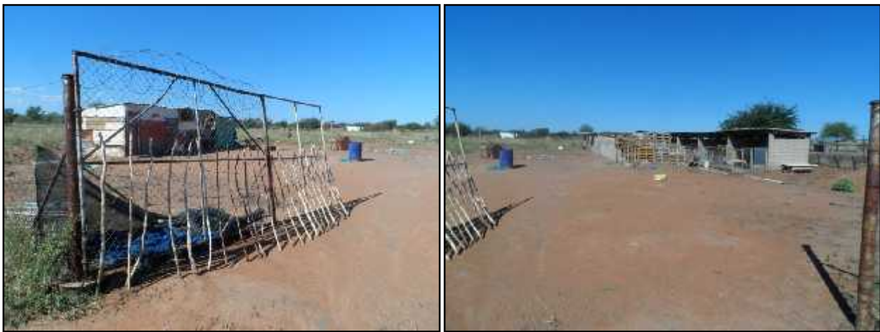
Figure 16-STIN-6, 2 residential shacks (left) and piggery structure (right)
