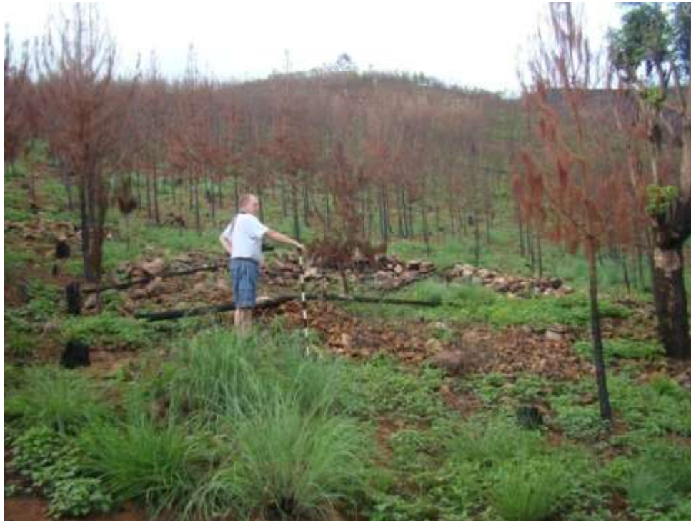
Fig. 154: This unit is located north of the graves (B35B), and is deteriorated and damaged by plantation activities. It is situated on a slope.
