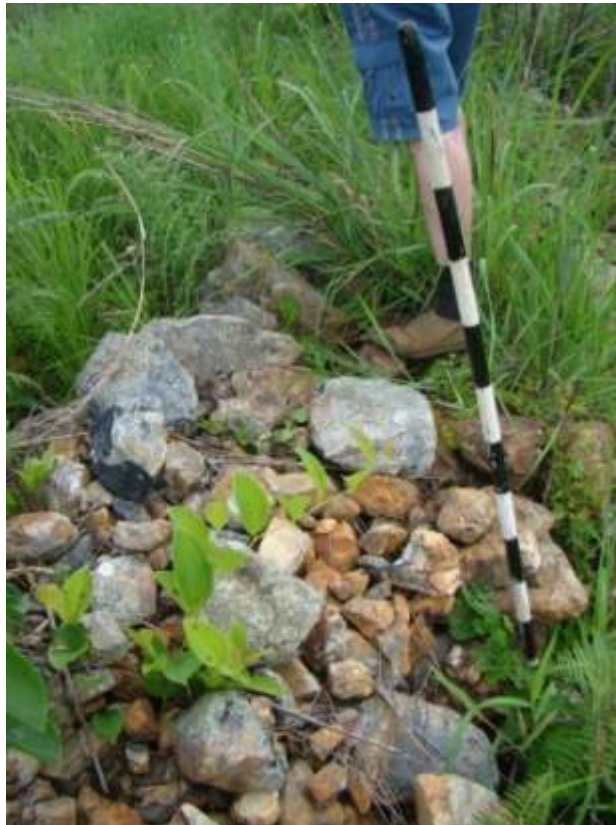
Fig. 153: Detail of the wall in this section.
