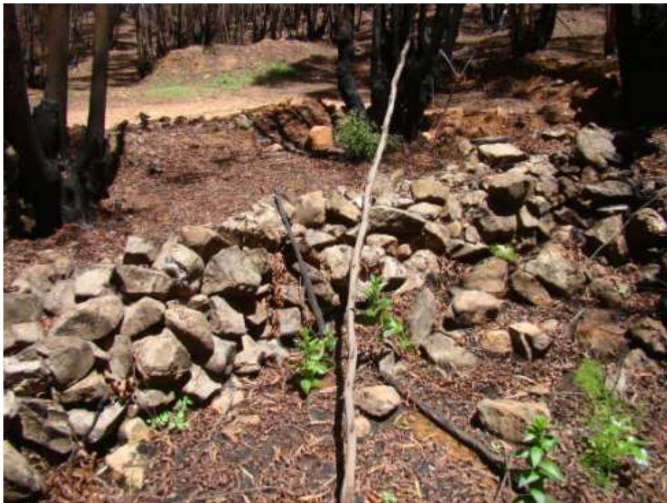
Fig. 109: The walls are in a fairly good condition and approximately 800mm high in sections.
