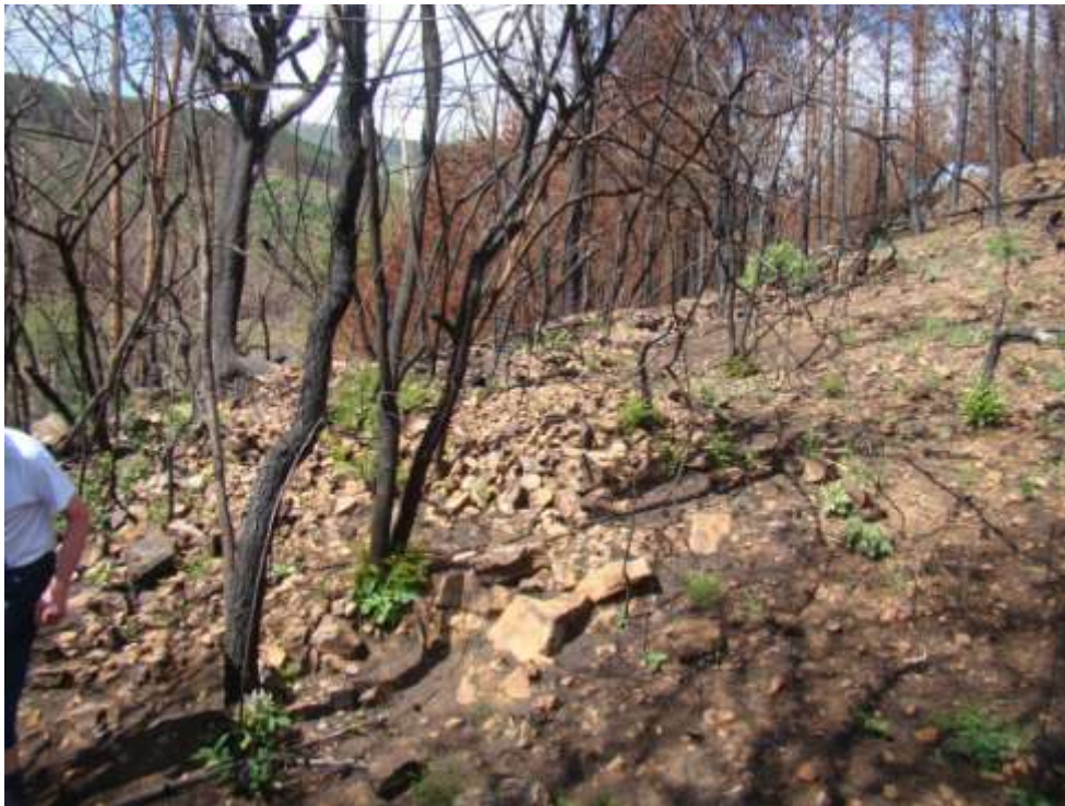
Fig. 197: The walls on the slope are mostly extremely deteriorated. Natural vegetation is seen in this section.
