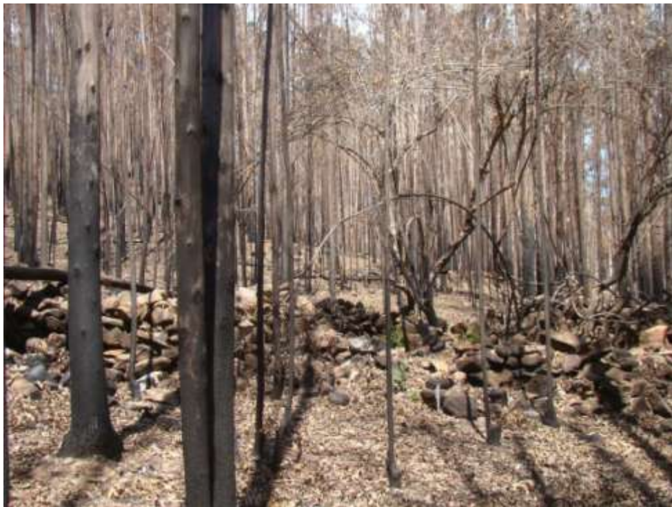
Fig. 210: 4 x units which are interlinked with walls. There are terrace walls and tracks below (north).
