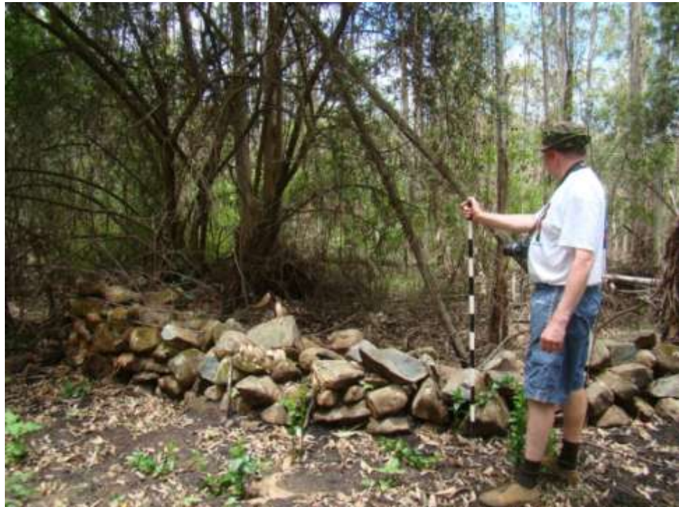
Fig. 143: A small section which is still in good condition.
