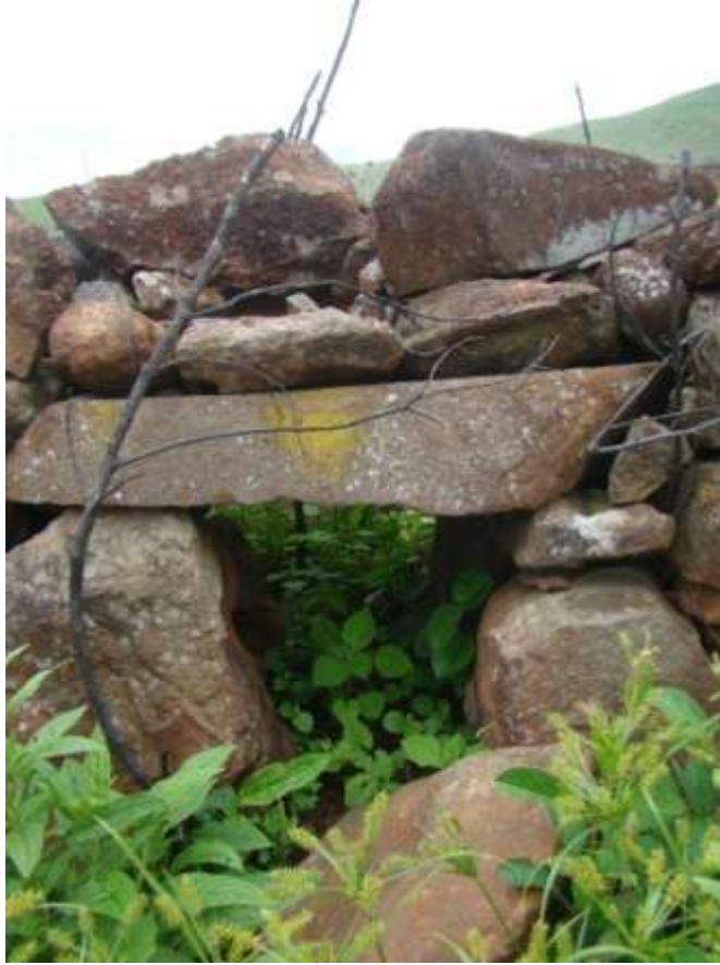
Fig. 229: Entrance opening with a stone lintel.
