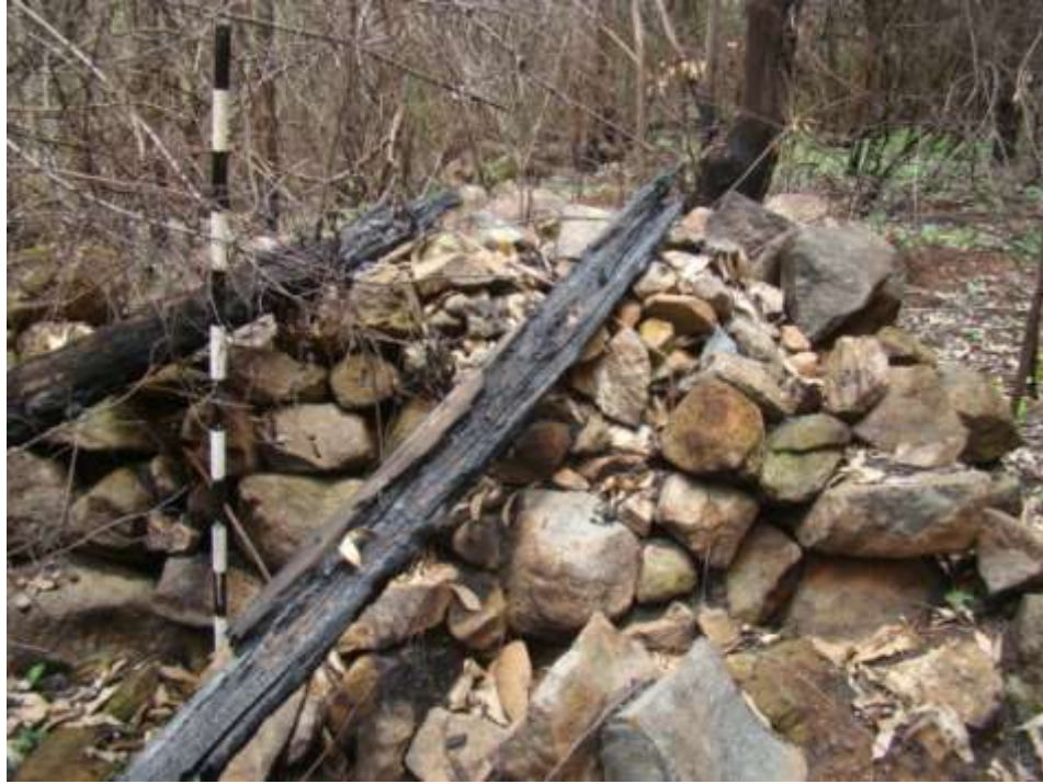
Fig. 123: Detail of the wall of the sheep kraal.
