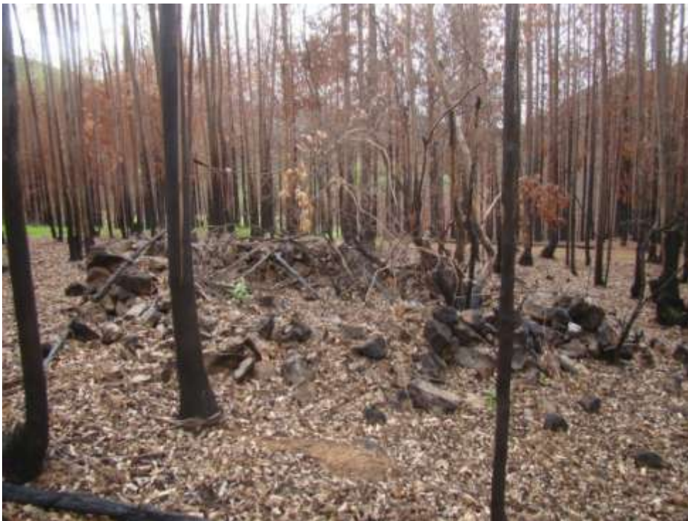
Fig. 192: Another stone wall which is damaged by vegetation.
