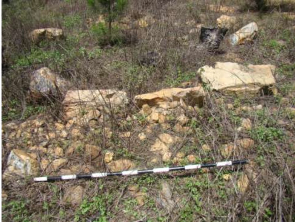
Fig. 12: Terrace walls which have been damaged by a road between compartments A12 and A13.
