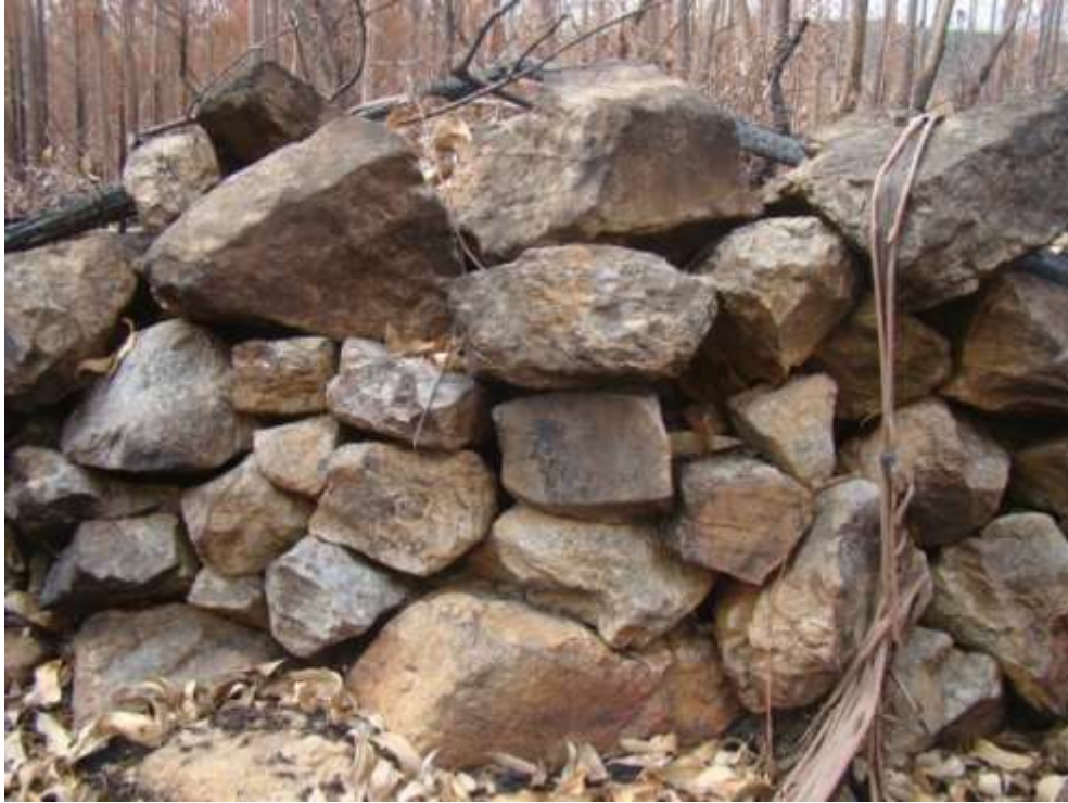
Fig. 193: An example of the walls.
