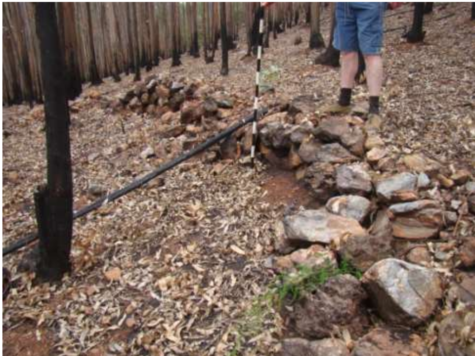
Fig. 147: Some of the terrace walls.
