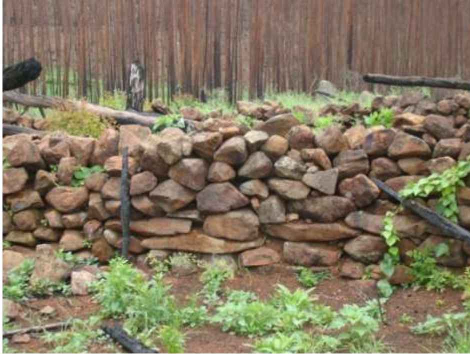
Fig. 233: The walls of the enclosure are still in a good condition.
