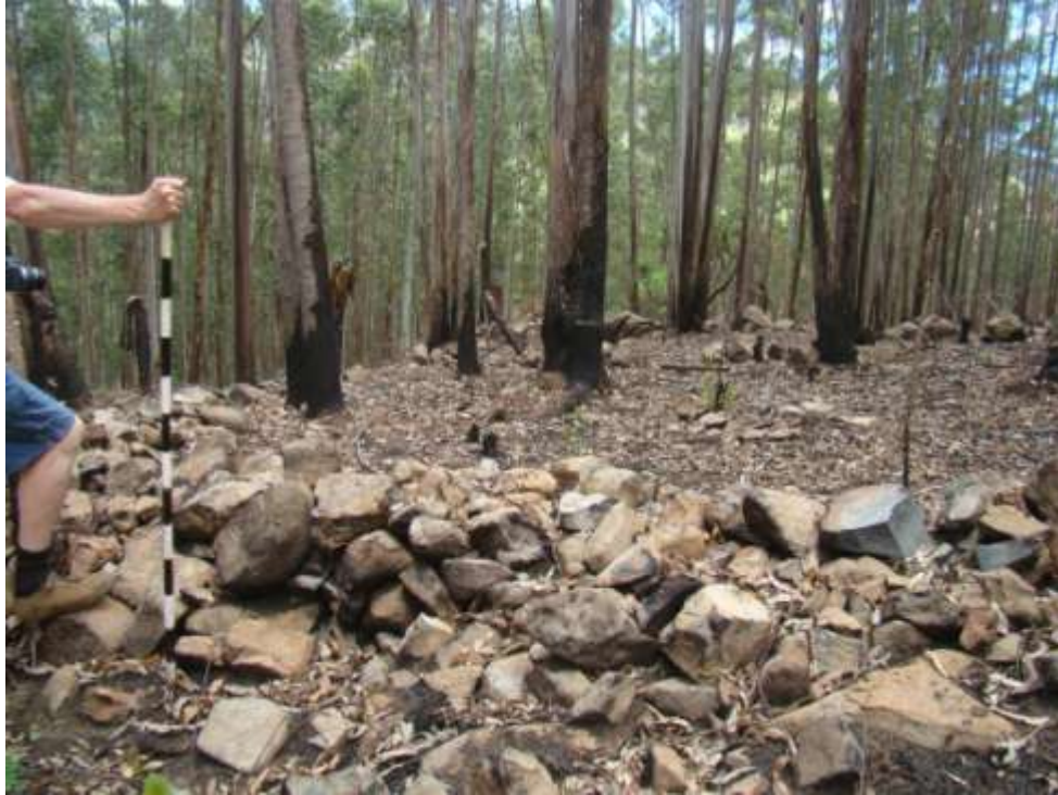
Fig. 142: The units down the southern slope are badly deteriorated.
