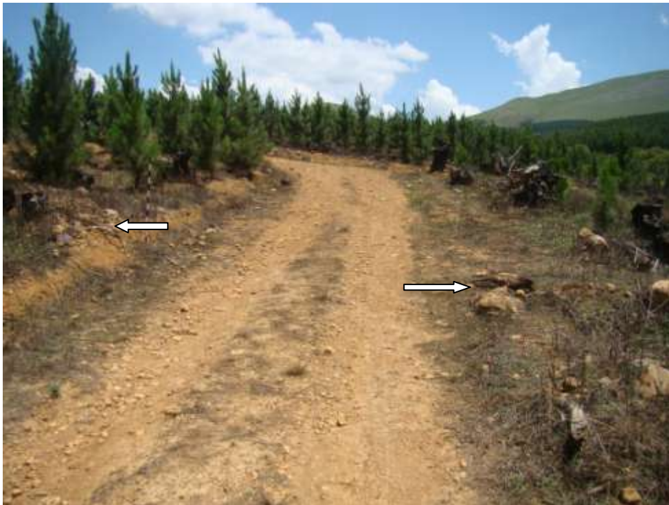
Fig. 13: Terrace walls which were damaged by road activities are visible on both sides of the road.
