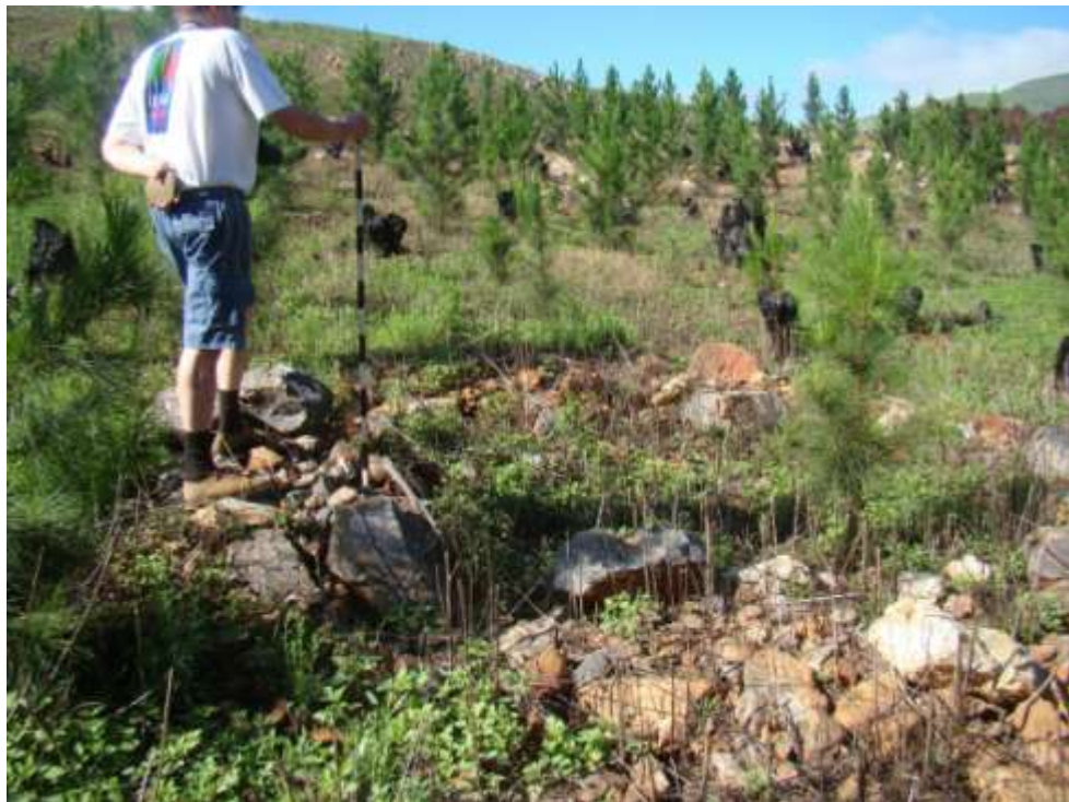
Fig. 98: Another deteriorated unit in section A21.
