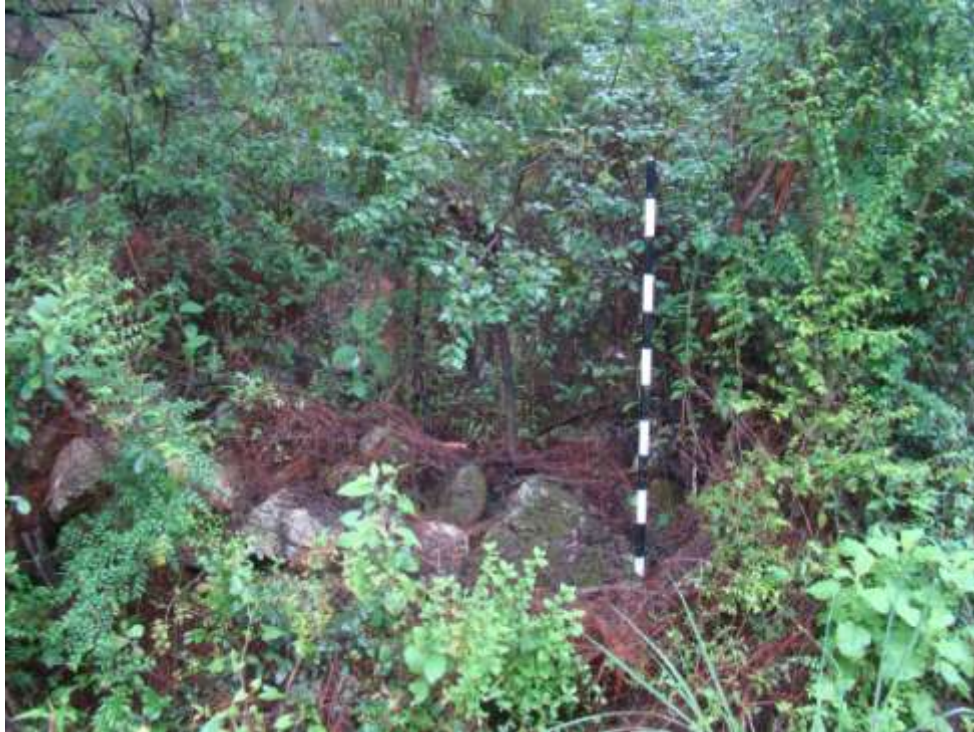
Fig. 57: A low wall which is overgrown with vegetation. This unit is damaged by road activities.
