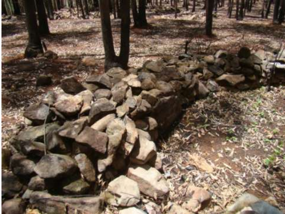
Fig. 114: Detail of the condition of some of the walls.
