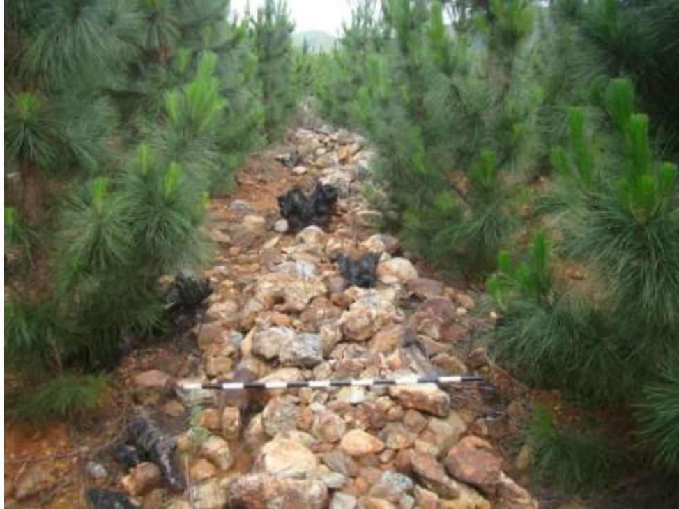
Fig. 46: A cattle track is deteriorated and run down but was approximately 1200mm wide.
