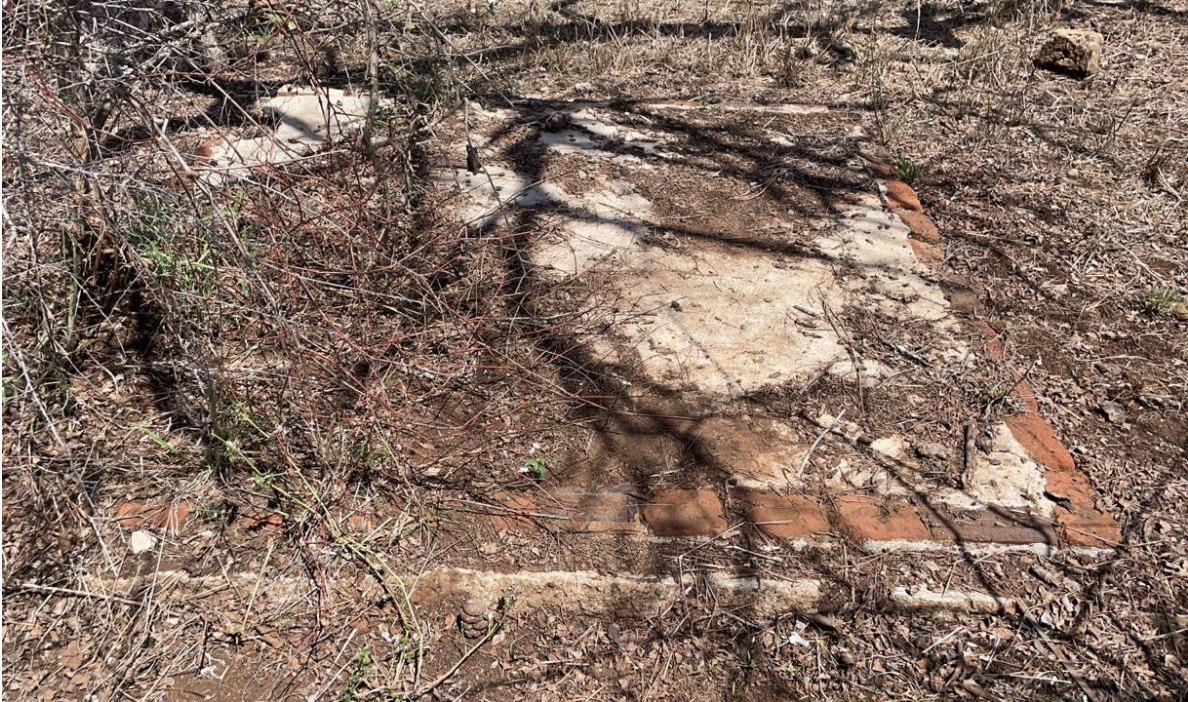
Fig. 13: A concrete & brick foundation in the vicinity of the structure.
