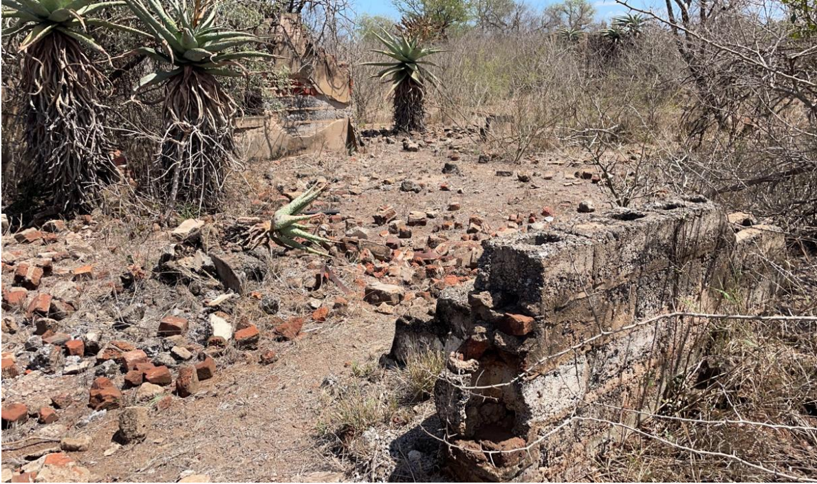
Fig. 11: The recent structure (house) was built with a large concrete as well as smaller baked bricks, and possibly dates back to the 1960's.
