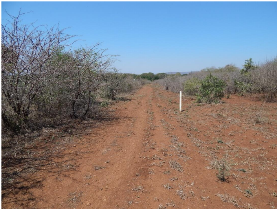
Fig. 6: The pipeline facing east.
