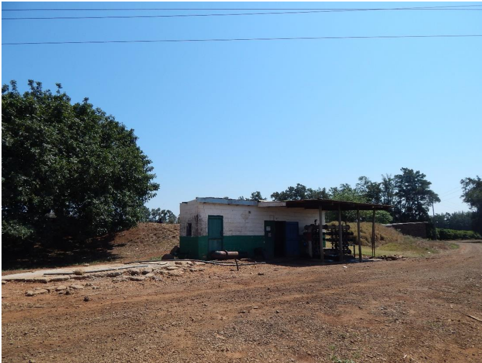
Fig. 28: One of the pumphouse structures on the farm next to a dam.
