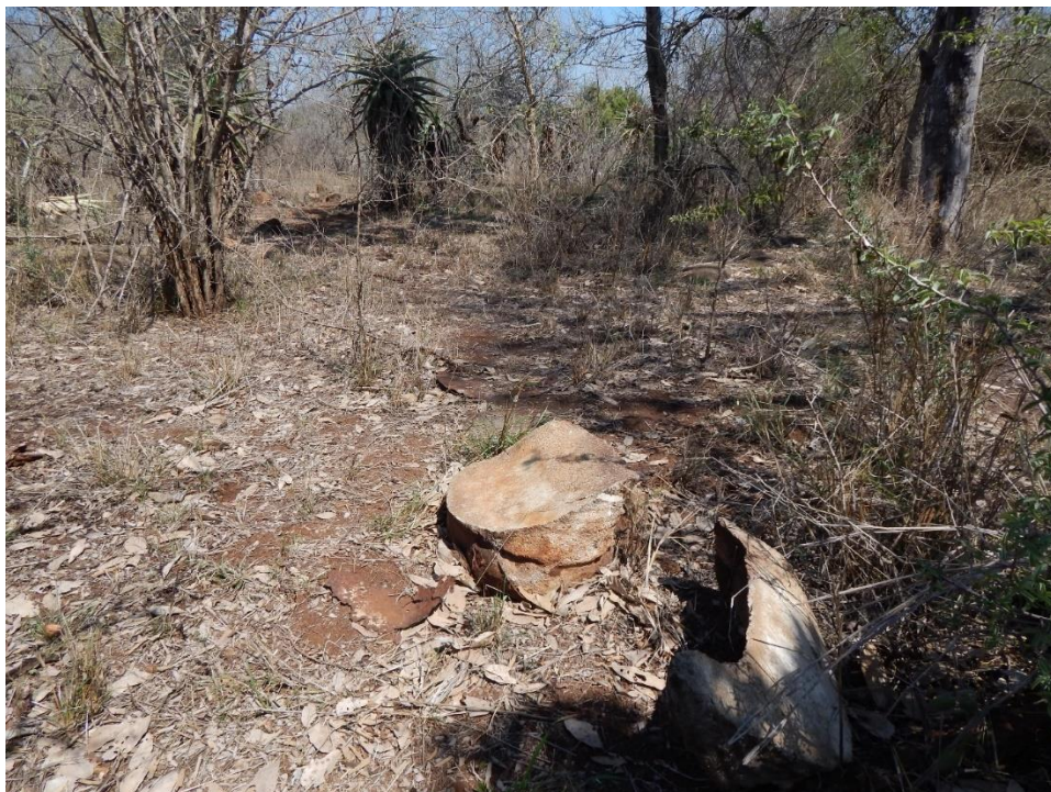
Fig. 14: Concrete and rusted metal pieces were observed closer to the Ngweti River.
