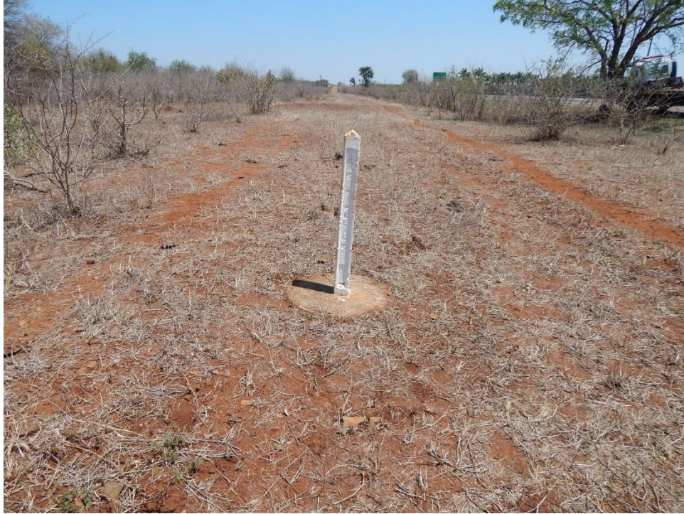
Fig. 5: A pipeline (SASOL) is located within the servitude area next to the N4 all along the northern border. View facing west.
