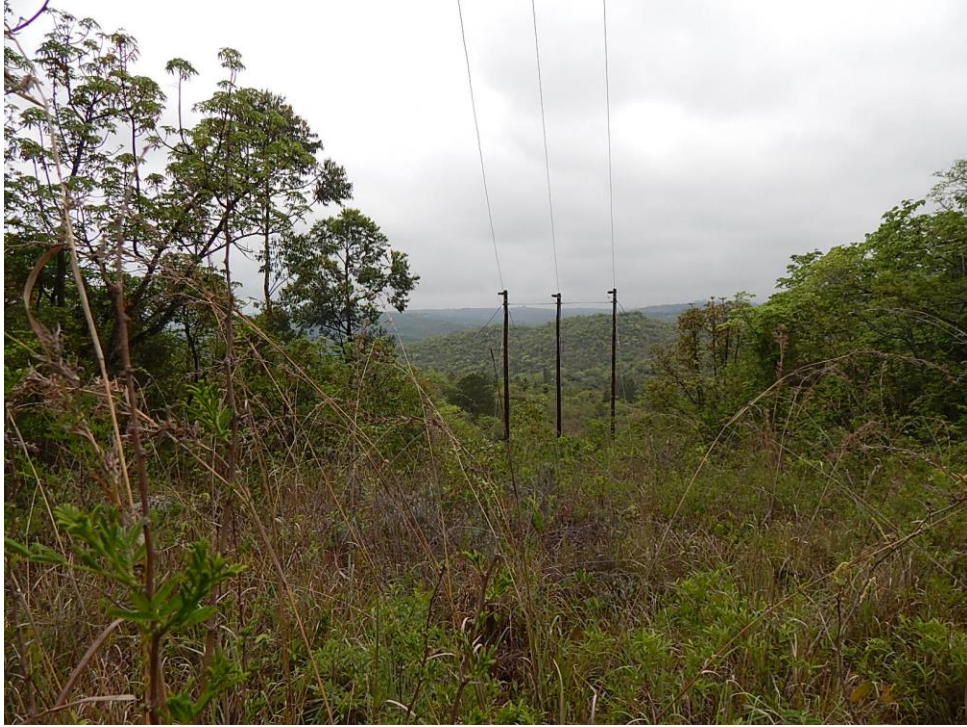
Fig. 3: The ESKOM power line was followed to access this dense area.
