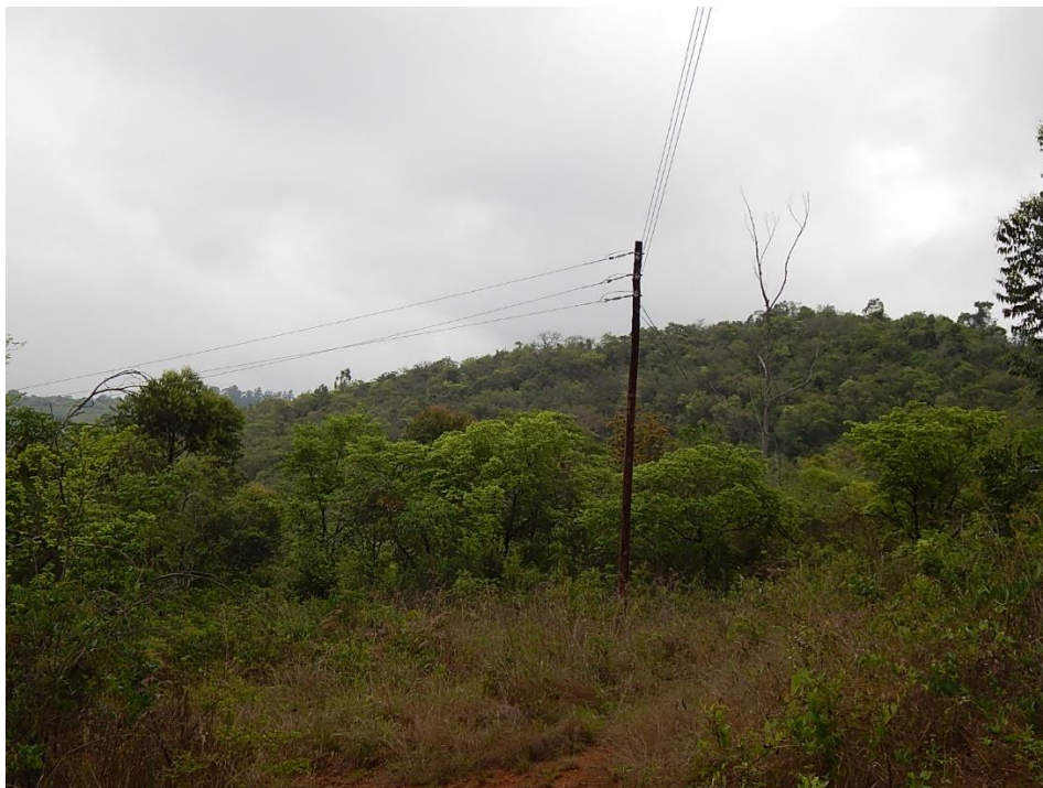
Fig. 2: An Eskom power line forms the southern boundary of section A.
