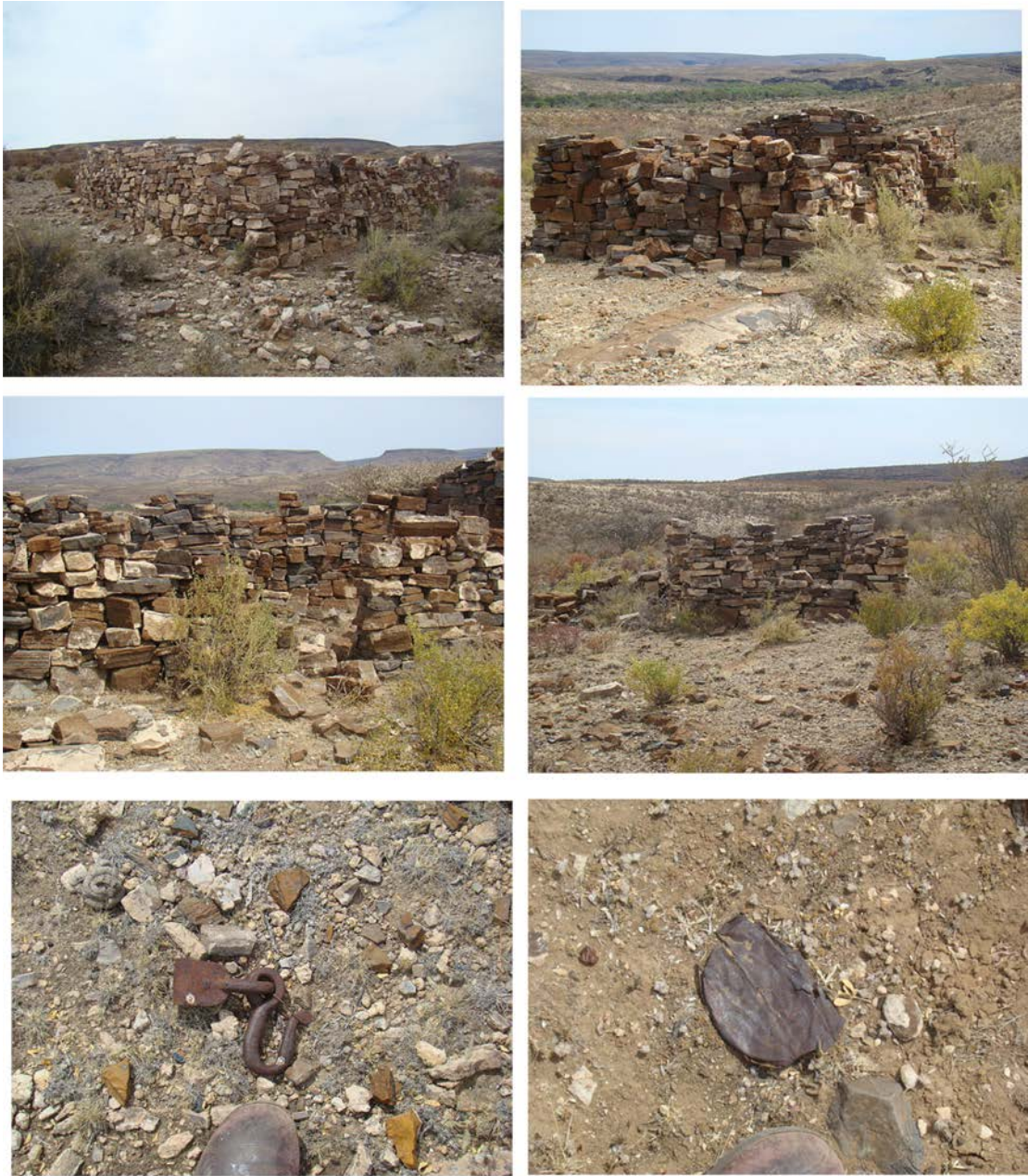
Figure 22. Site #121-164. Stone-walled ruins at Kliphuis 29. The site is associated with the asbestos mining industry that prevailed in the region more than a hundred years ago.
