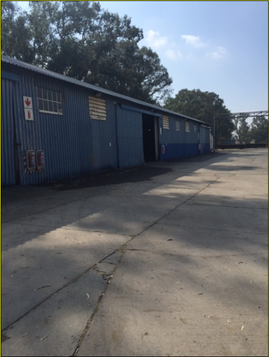
Figure 9. Maintenance building dating from 1957
