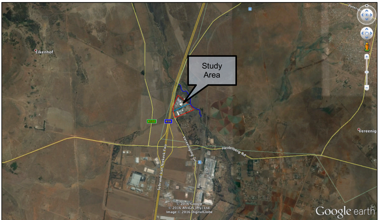
Figure 4. Aerial View of Proposed Expansion of the Tissue Manufacturing Capacity at the Twinsaver Klipriver Operations Base, Gauteng Province
