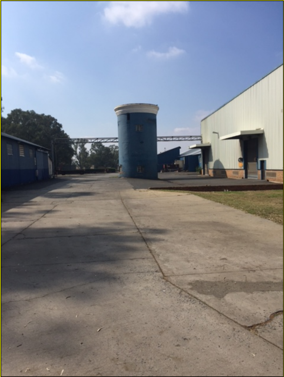
Figure 8. Farm silo dating from early to middle 1900's (not to be altered)
