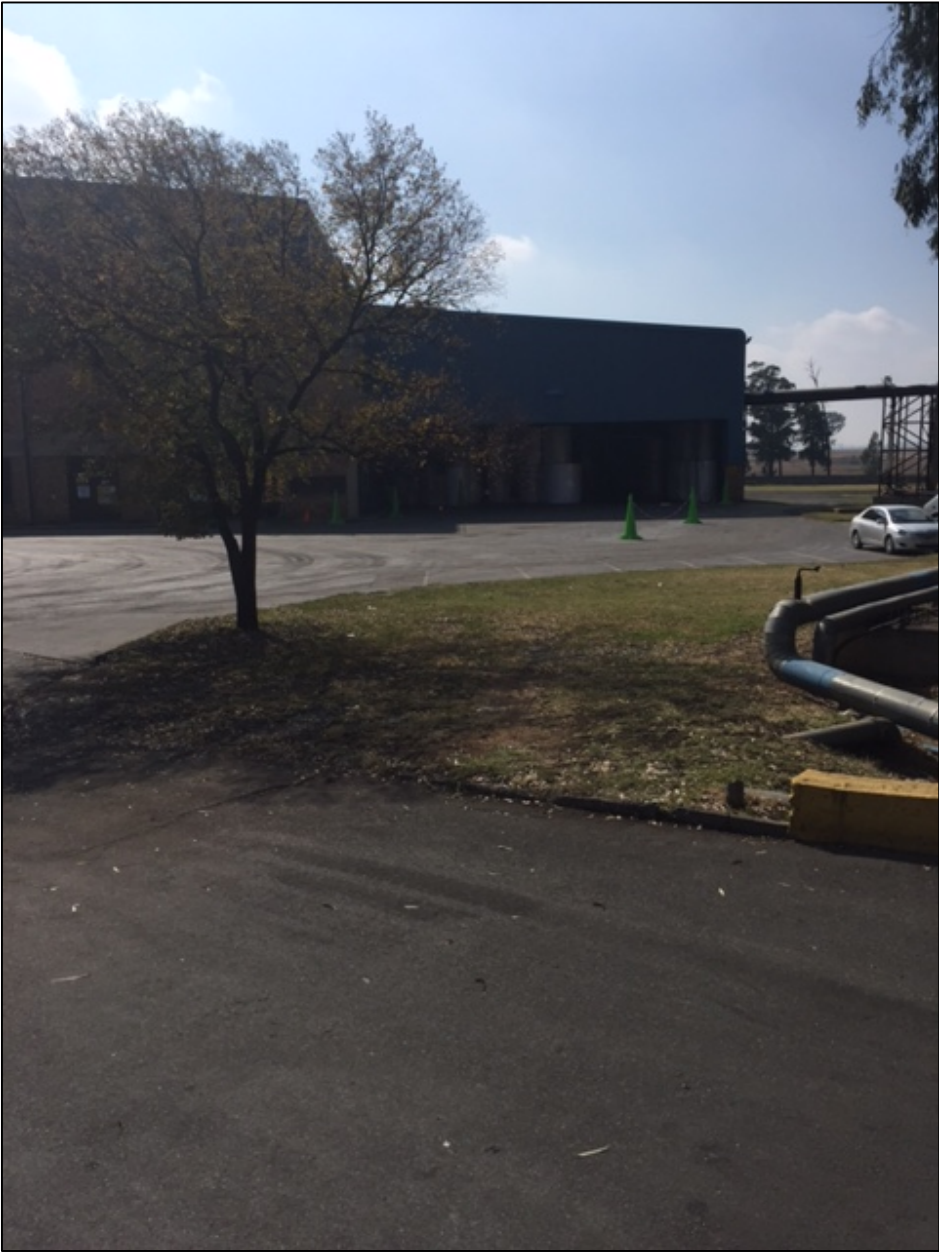
Figure 11. Building to be altered dating from 1991
