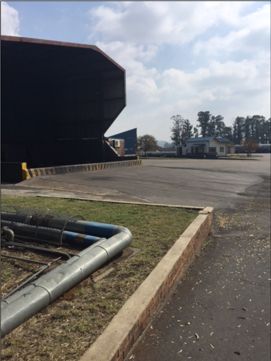
Figure 12. Bond store dating from 1976 (not to be altered)
