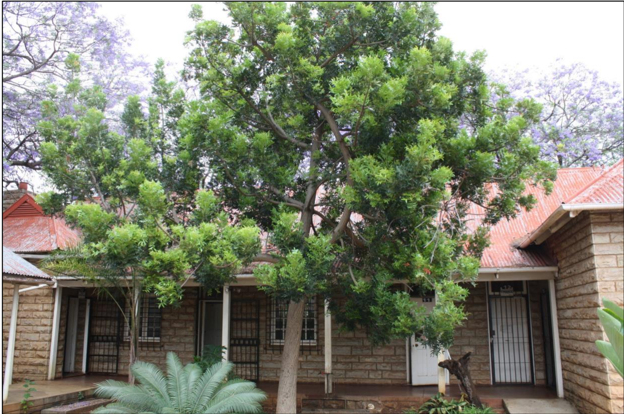
Figure 11. Mokopane Police Station Sandstone Building
