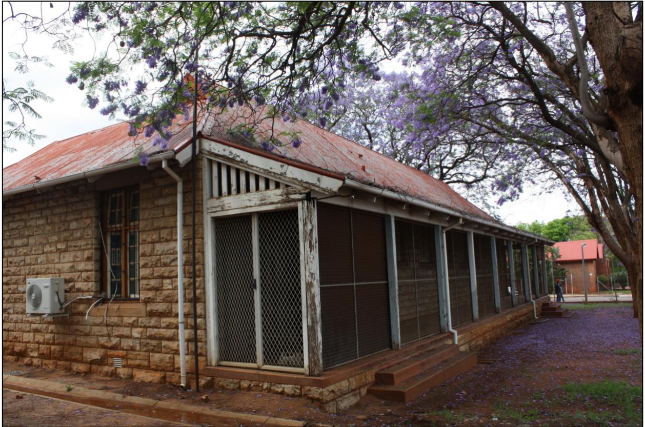
Figure 16. Mokopane Police Station Sandstone Building
