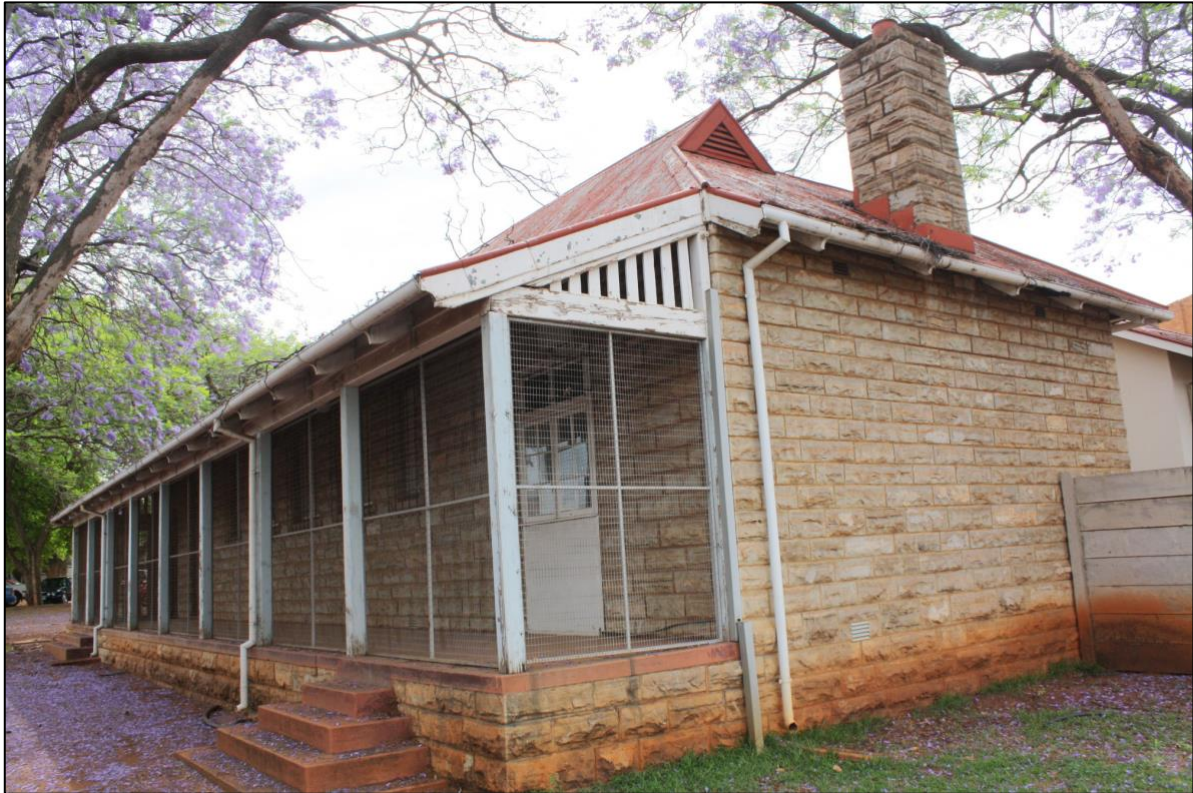
Figure 12. Mokopane Police Station Sandstone Building
