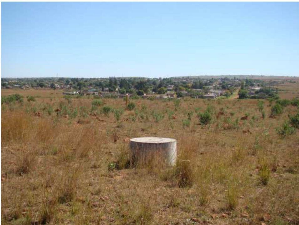
Fig. 4: The north-south pipeline at point 7, facing north.
