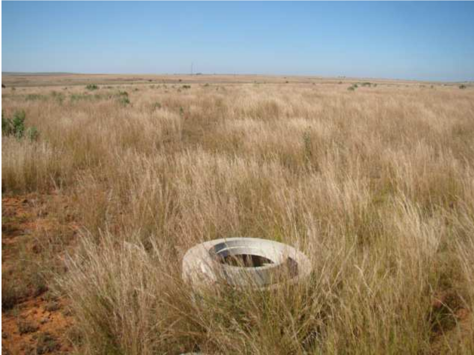
Fig. 5: North-eastern section. The east-west pipeline facing from east (near point 1) to west.
