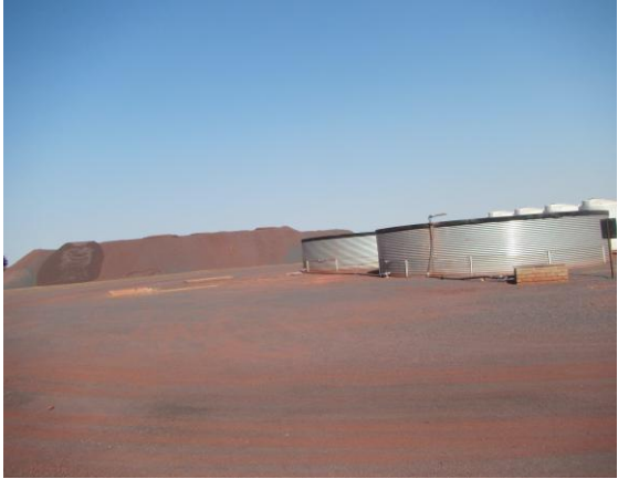
Quarry and Road construction activities .
