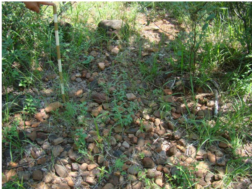
Fig. 18: Another recent stone foundation which is almost entirely deteriorated.
