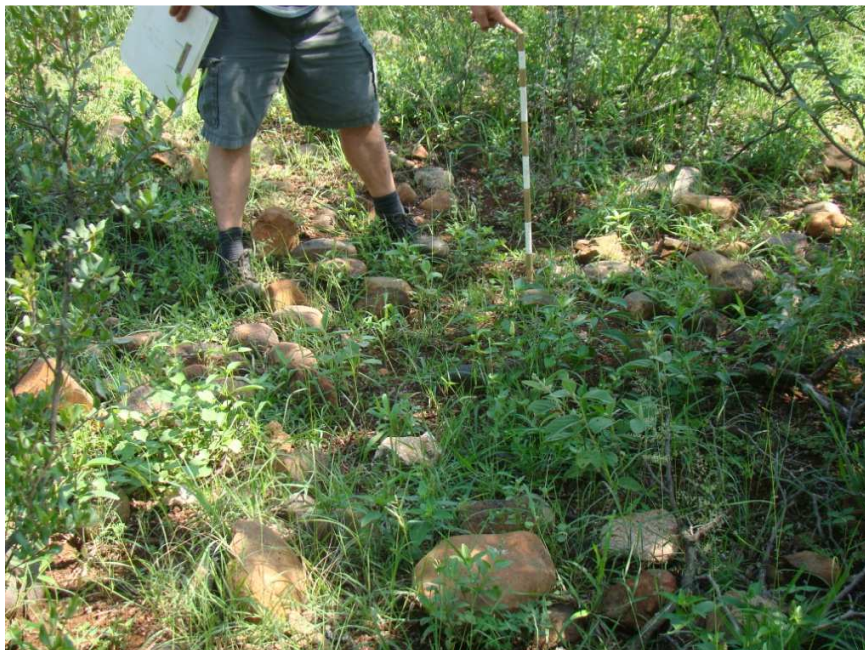
Fig. 14: A recent stone foundation or terrace wall.
