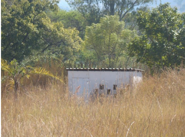
Fig. 9: The Pump house.
