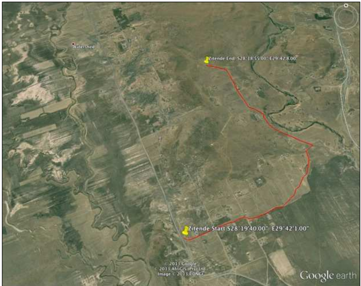
Figure 2. Aerial view of proposed upgrade
