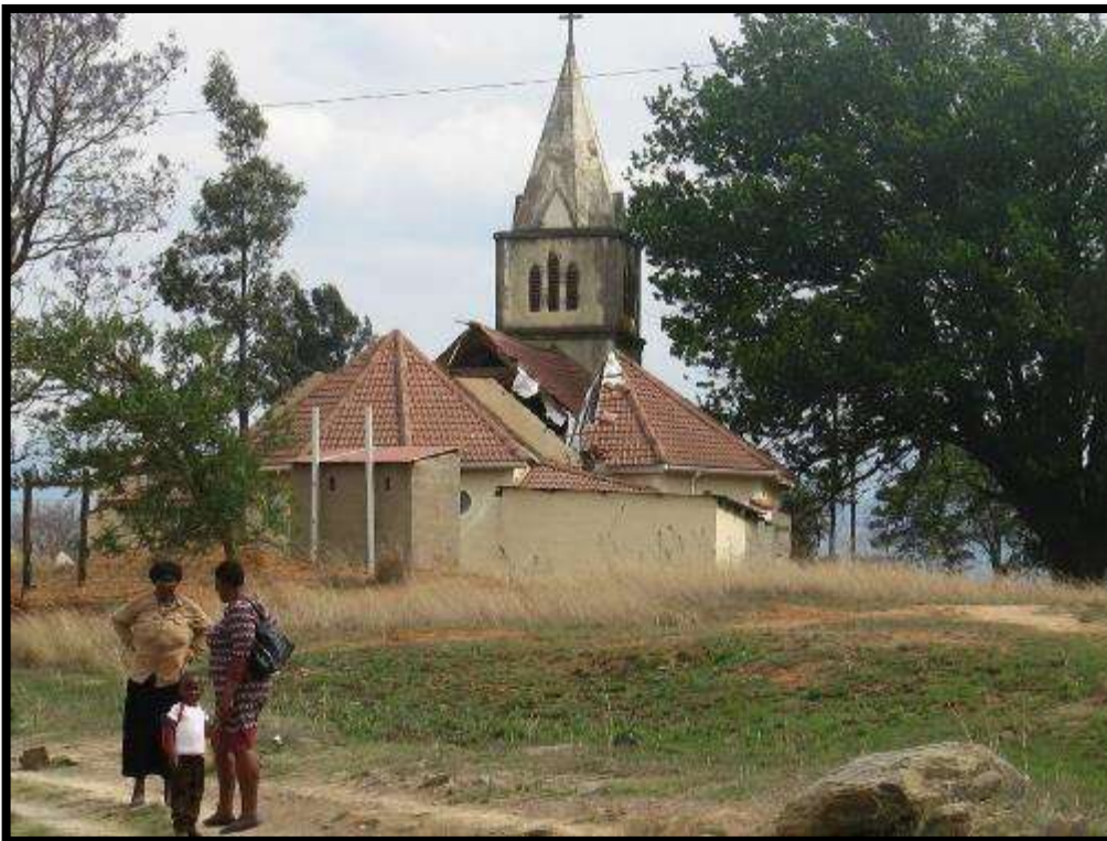
Figure 8. The Emmaus Mission Station and Church is situated approximately 1.5km from the start of the footprint. It is not threatened by the proposed development and there is no need for mitigation. The old church buildings have fallen in disrepair.
