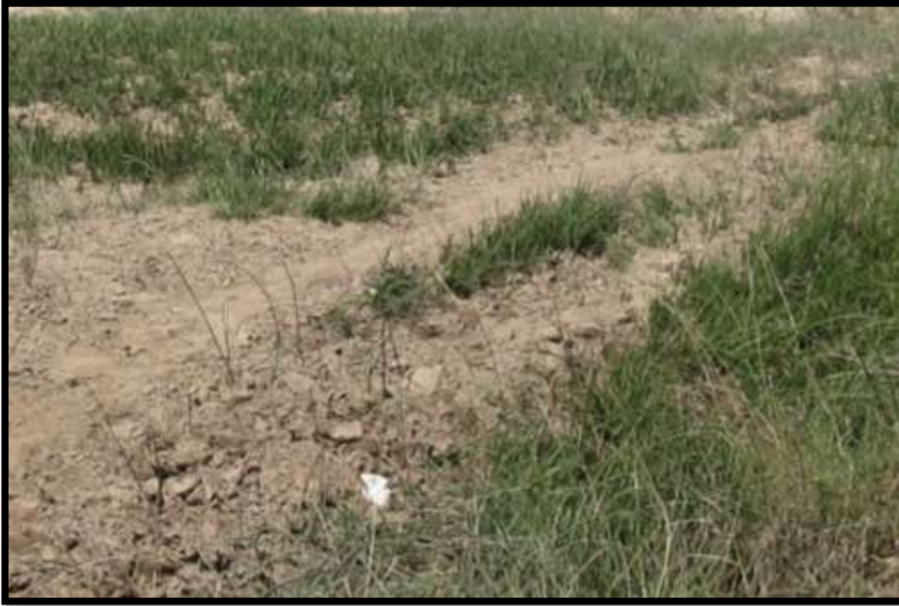
Figure 5. The existing mud track earmarked for upgrading photograph taken near the start of the road.
