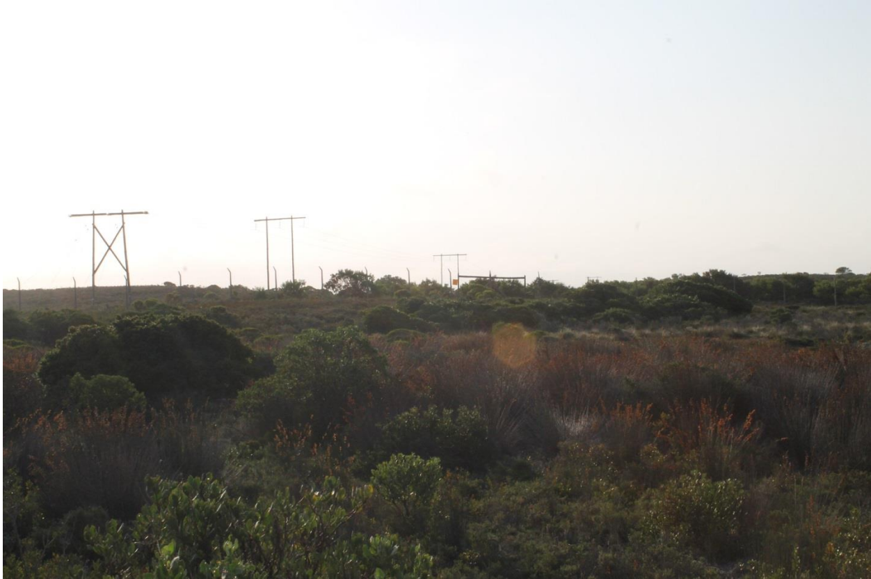
Figure 5 The end of the existing 66 kV power line at Arniston just inside Denel property. The last 1.5 km consists of densely vegetated un-transformed land and seasonal wetland..
