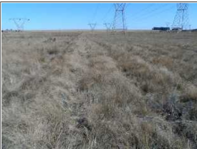
Figure 13- Grass cover under powerlines
