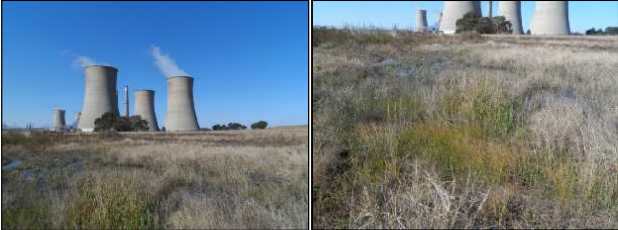
Figure 12- Ground water seepage
