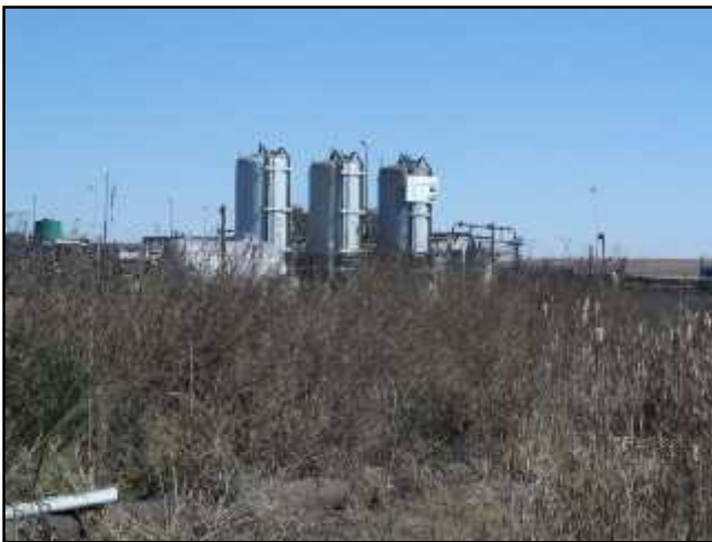
Figure 9 - Storage tanks or cylinders
