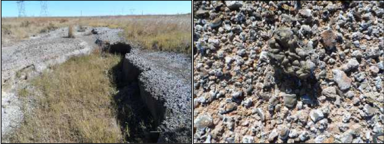
Figure 14- Ground leaching, showing evidence of ash and burnt material - typical waste dump site material.
