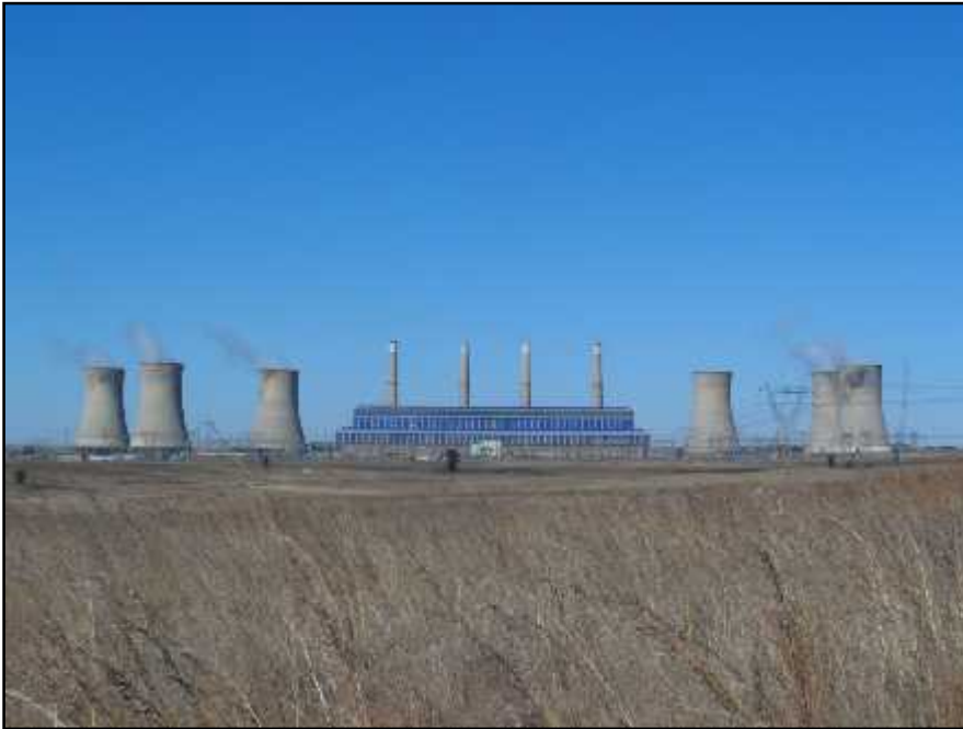
Figure 3 - Camden Power Station - note the flatness of the landscape
