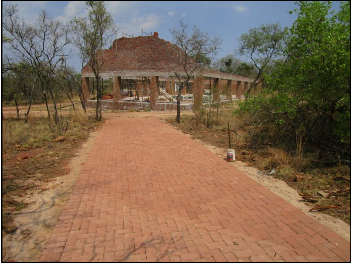
Figure 10. View of an incomplete building, which as the others clearly indicated that all activities were ceased because of the lack of authorisation for the development.
