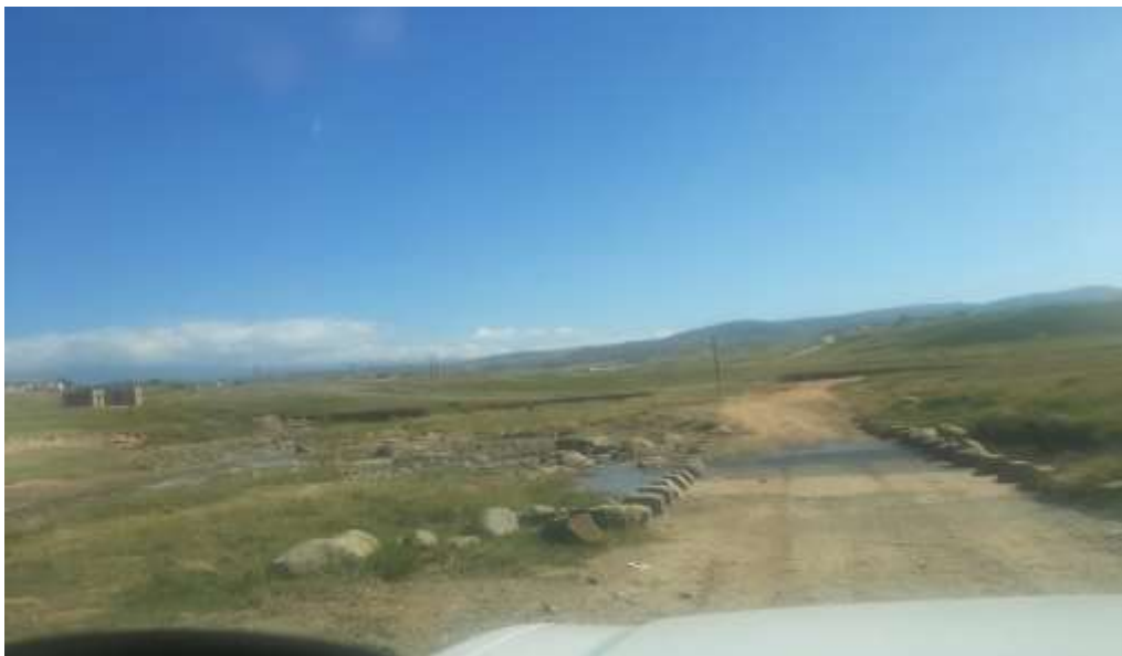
Figure 6: A small bridge the proposed road will cross over.
