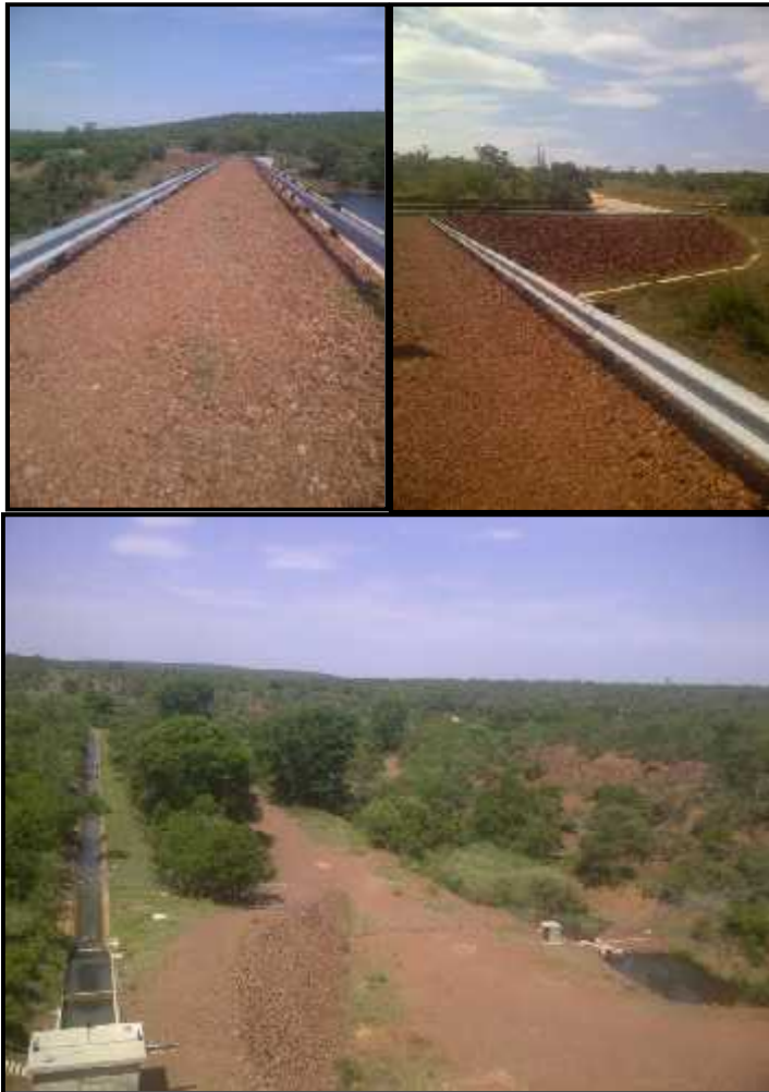
Figure 9- Dam wall and discharge Rust De Winter Dam
