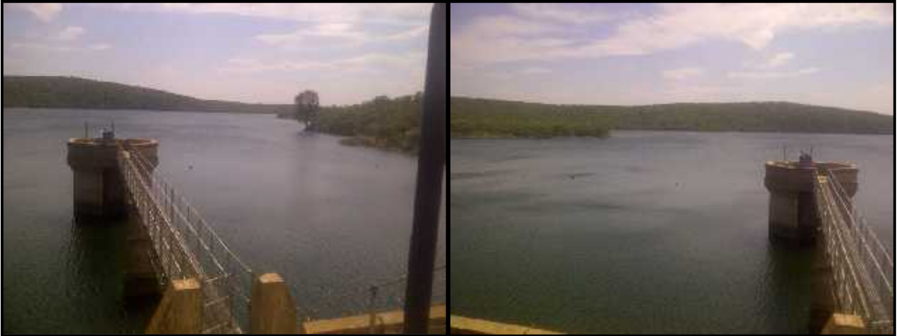
Figure 8- General view Rust De Winter Dam
