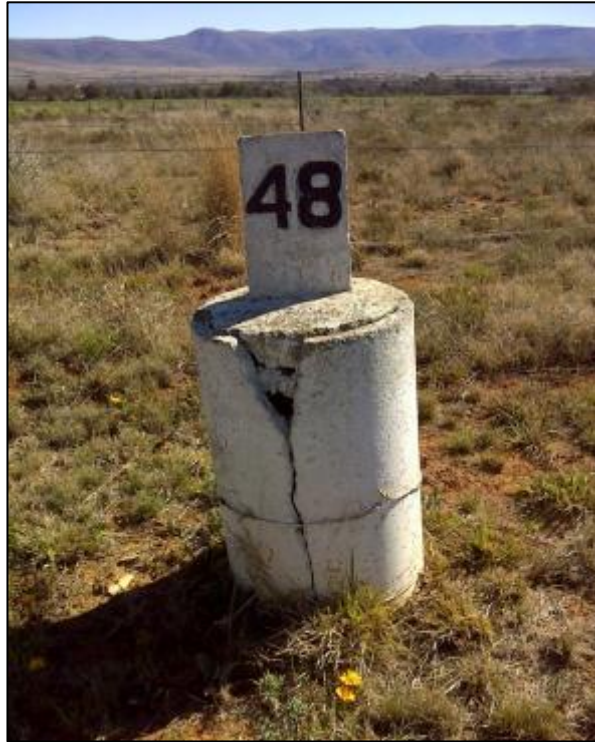
Figure 2-5: Structure situated at S1 5km north of the Riet River Bridge.
