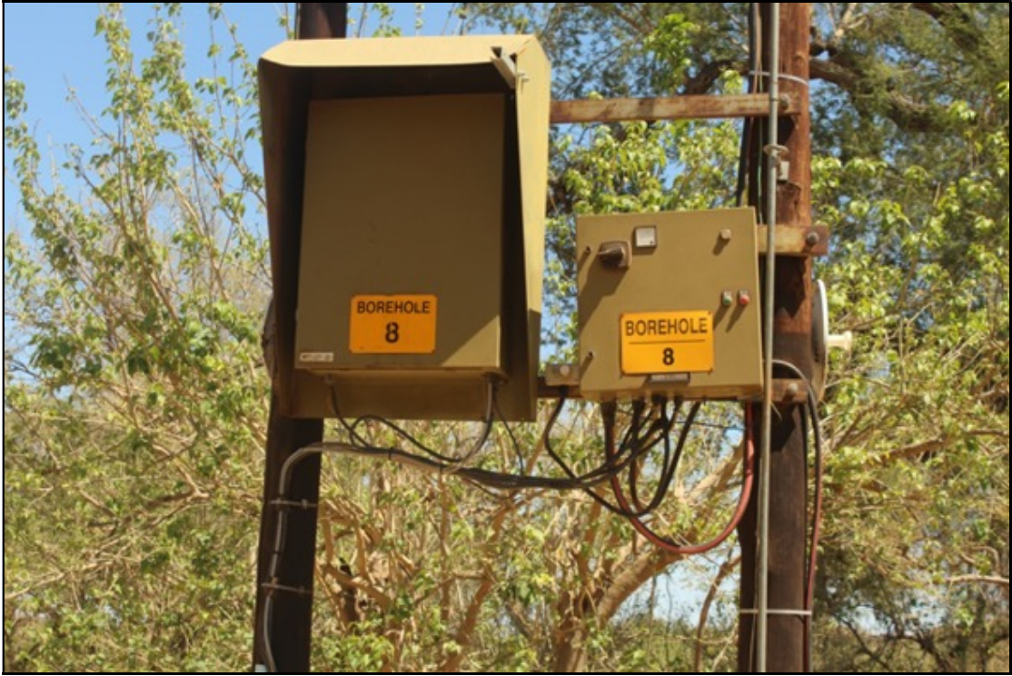
Figure 11: Borehole No:8 Switching station
