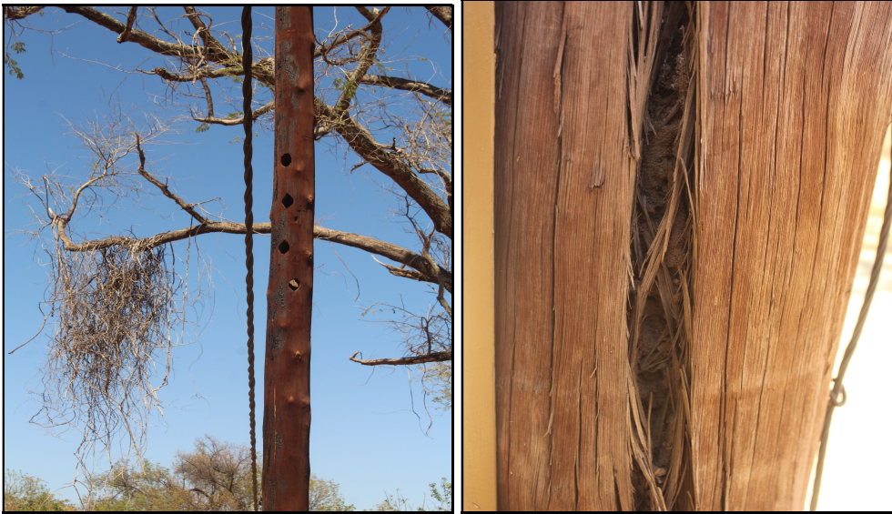
Figure 2: Damaged powerline poles
