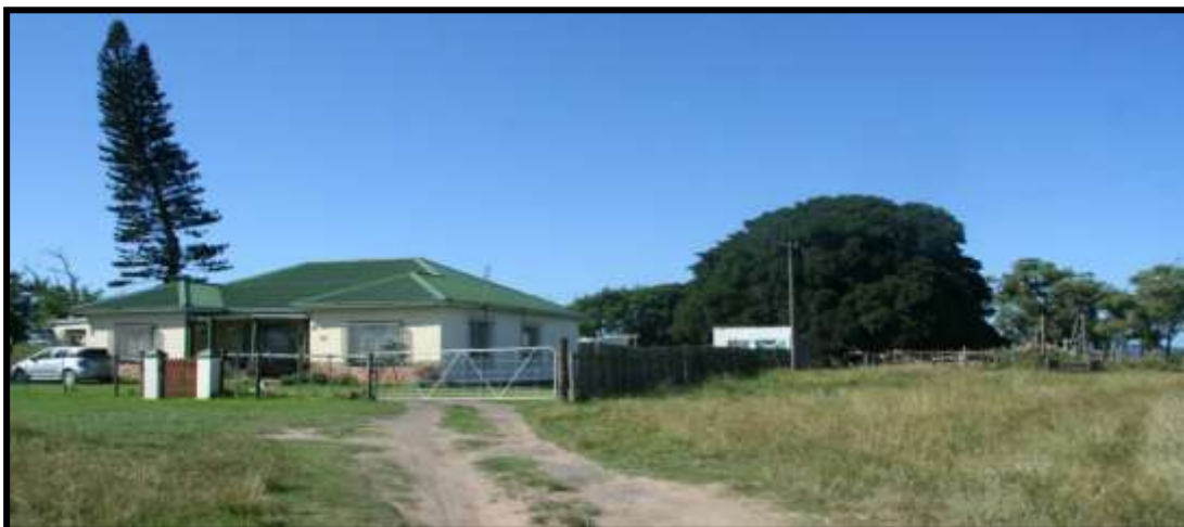
FIG. 7: FARMHOUSE AT CDW-F1
