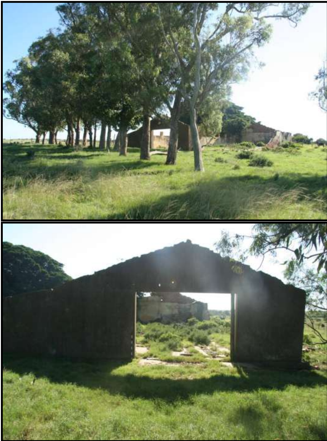
FIG. 8: FARMHOUSE AT CDW-F1
